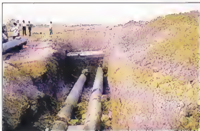
Underground pipeline while laying
