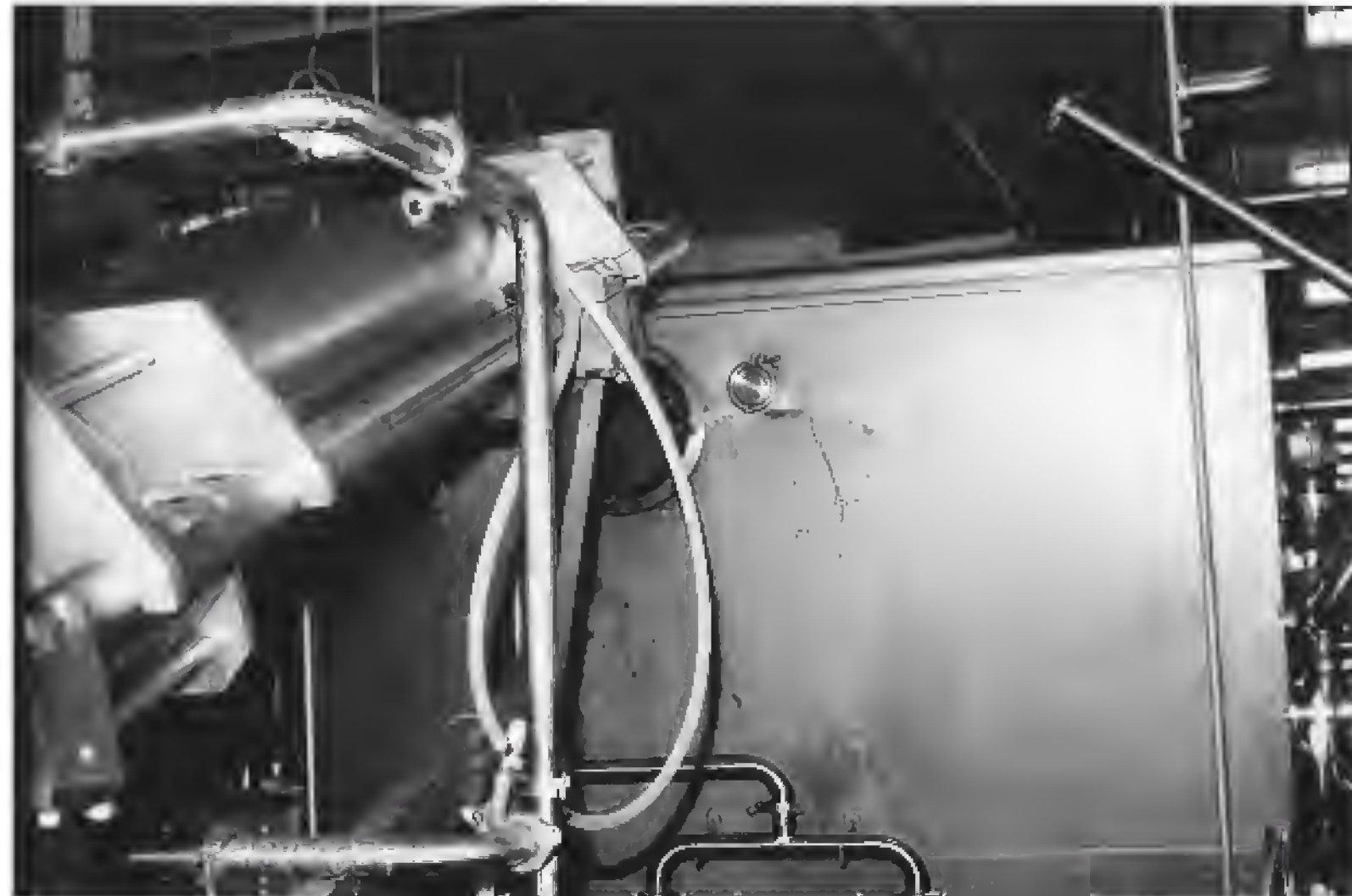
Figure 3 Butter is delivered from the turret end of the continuous churn into a covered silo.
