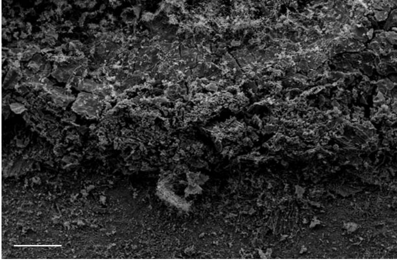
Fig. 5. Deterioration of a concrete block that was exposed to fungal weathering for 2 years in an experimental microcosm (M. Fomina and G. M. Gadd, unpublished). Cracking is evident, as well as an extensive hyphal net over the surface. Bar, 200 \mu\text{m} .
