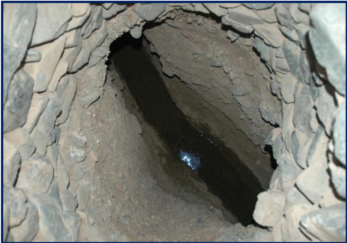
A qanat , showing one of the characteristic wellhead accesses that facilitated construction, ventilation, and water extraction. The English word “canal” is derived from the classical Arabic word “qanat”. Picture source: John Baez.
