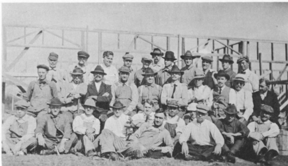
THESE CONFERENCE WORKERS BUILT THE BARN AND THE GARAGE.
