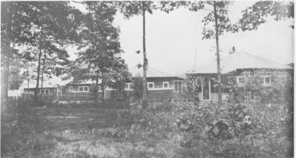
THE CLASS IN WOODWORK BUILT A TEACHER'S COTTAGE EACH YEAR.
