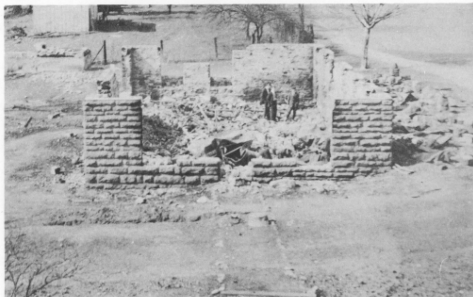
AFTER THE FIRE FEBRUARY 18, 1915
