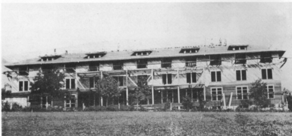
BUILDING THE WOMEN'S DORMITORY, 1917
