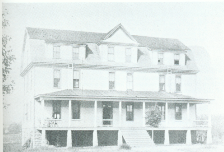
THE WOMEN'S DORMITORY AT SOUTHERN TRAINING SCHOOL
