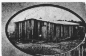
A temporary dormitory used by the boys. They often work until midnight including teacher and other freight in order to alleviate as much as possible their misery in each quarter. Many would not think of spending any time in such buildings.
