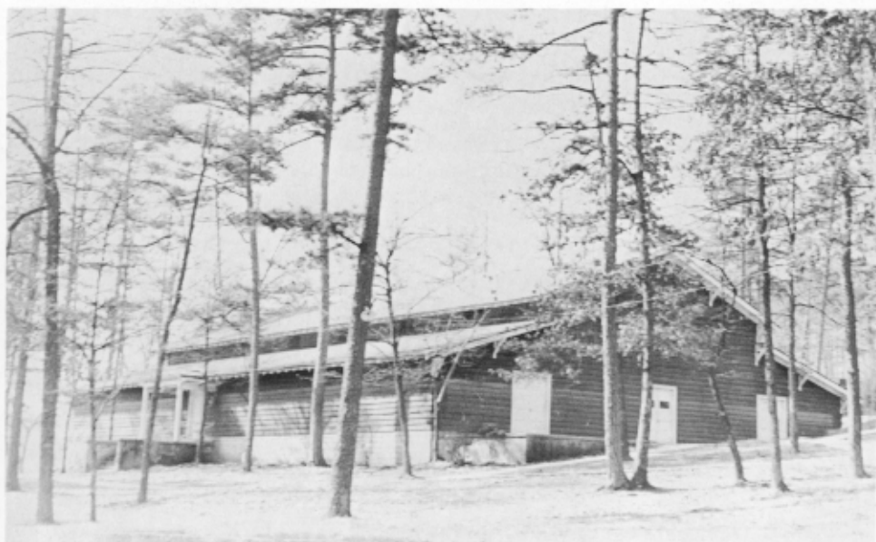
THE TABERNACLE BUILT IN 1934. NOTE THE WOODEN SHUTTERS IN PLACE OF WINDOWS; THE BUILDING WAS TWO-THIRDS ITS PRESENT LENGTH, AND THERE WAS NO VERANDA.
