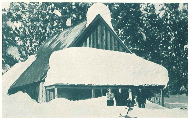
Many deep winter snows have tested the serviceability of the Sugar Pine used in this building in the Sierra Nevada of California.
