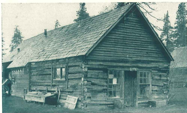
Another pioneer structure, the Olesen cabin, built of Sugar Pine in 1868 at Chester, California, in the high Sierra. Never painted or given any preservative treatment. Cabin sixty-five years old when photographed.
