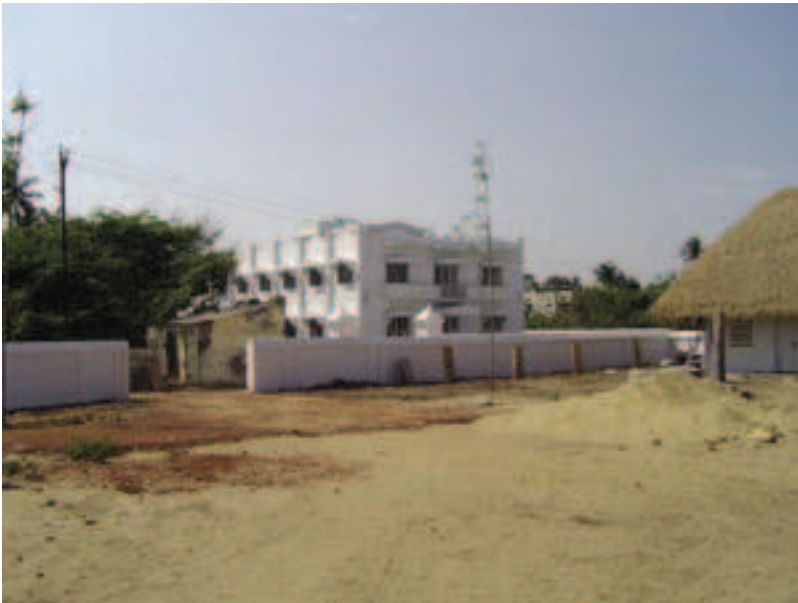
PLATE 1 4 Extension of dormitory of the bungalow, Tarangambadi
