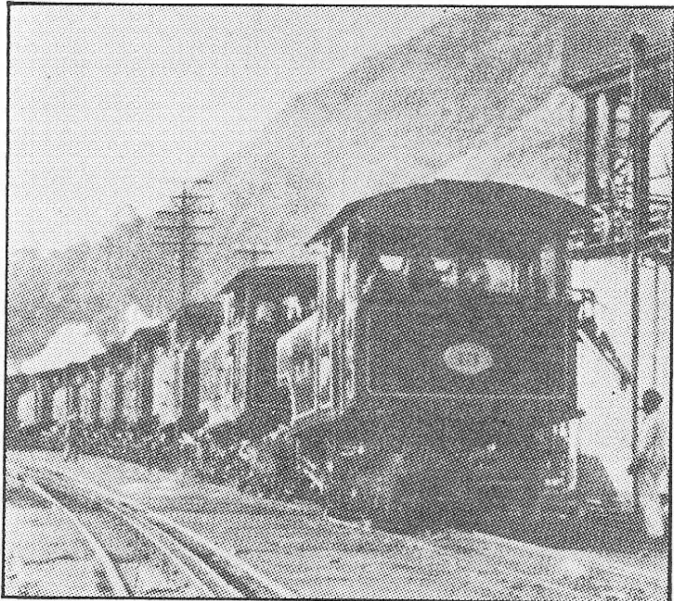
Boilers Set Level on the Incline
