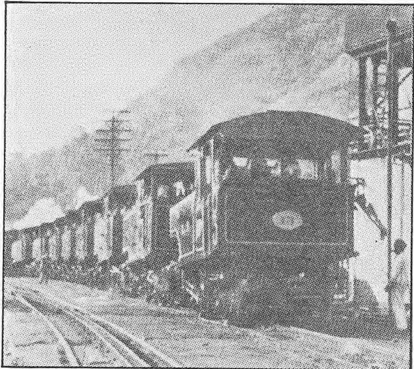
Boilers Set Level on the Incline
