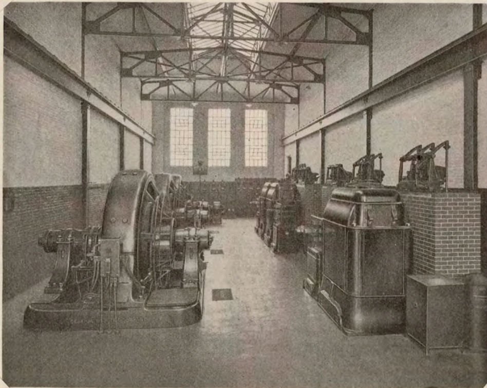
Fig. 7. Mt. Royal Substation of the Baltimore and Ohio Railroad
