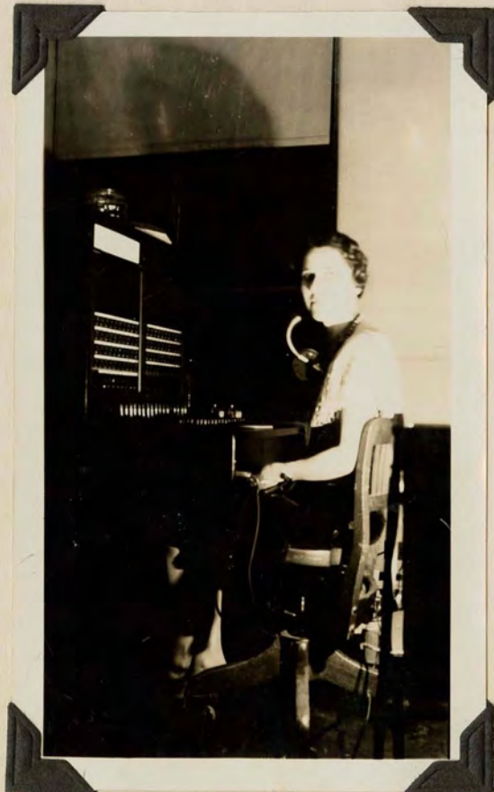
Private Branch Exchange Switchboard
