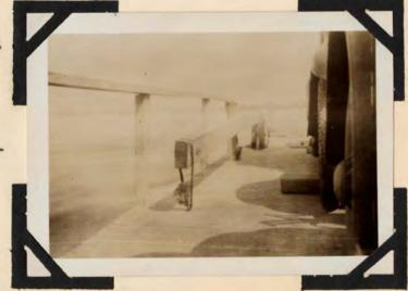
Constructed of heavy white oak planks secured cross-wise on four shorter battens, the gang board is obviously the limiting factor with regard to the individual loads which can be carried. Probably the heaviest single unit transported was a C. & P. Telephone Company line truck fully loaded with wire, the weight of which may have reached seven tons.
