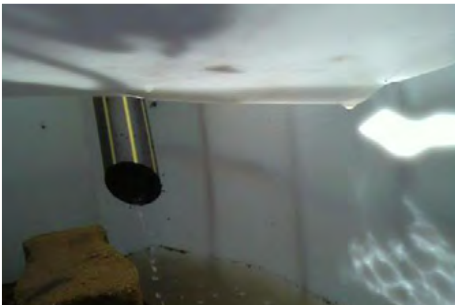
Water returning from bath adding aerations as it breaks the surface
