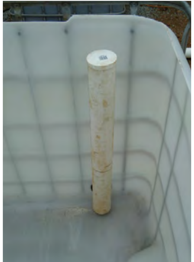
Standpipe surround to keep media away from the standpipe
