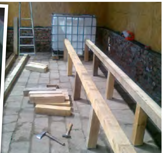
Heavy duty beams to support the growbed
