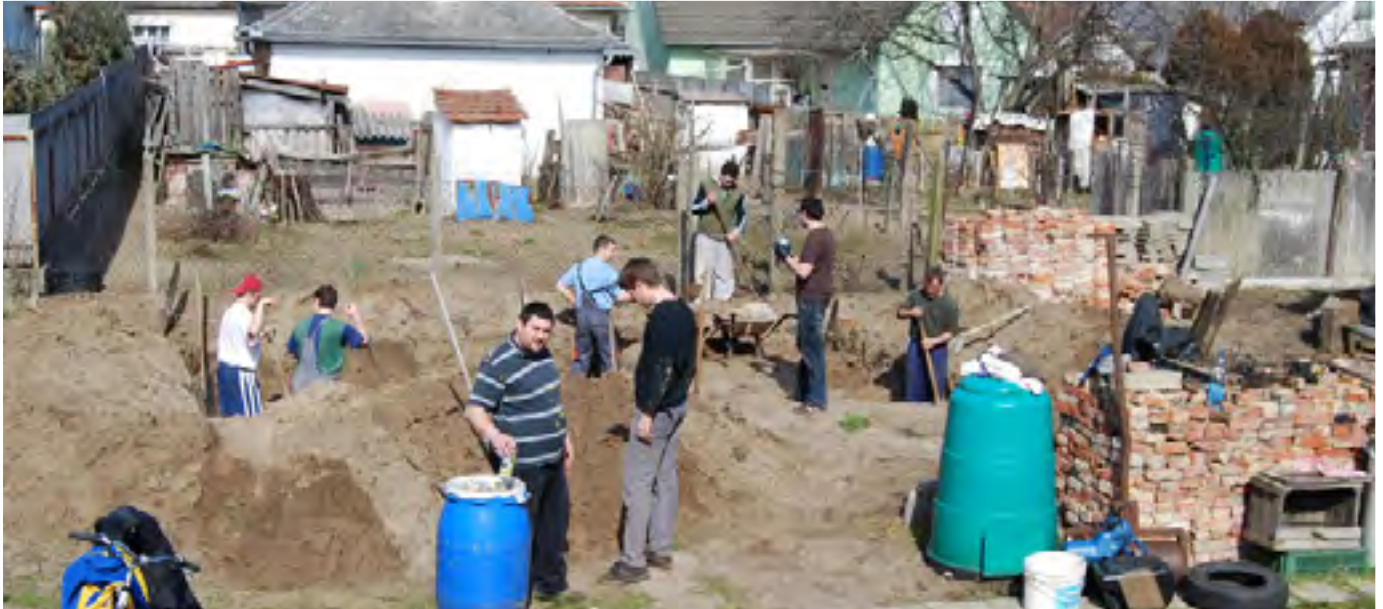
A busy worksite, it pays to have friends when there's lots of digging to do
