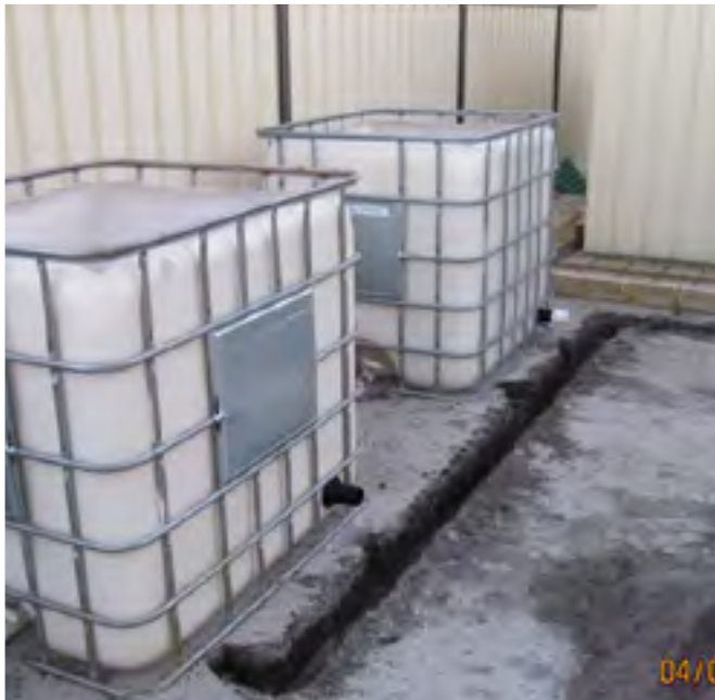
1st 2 IBC's in place with tank fittings installed and trenches dug ready for pipe work
