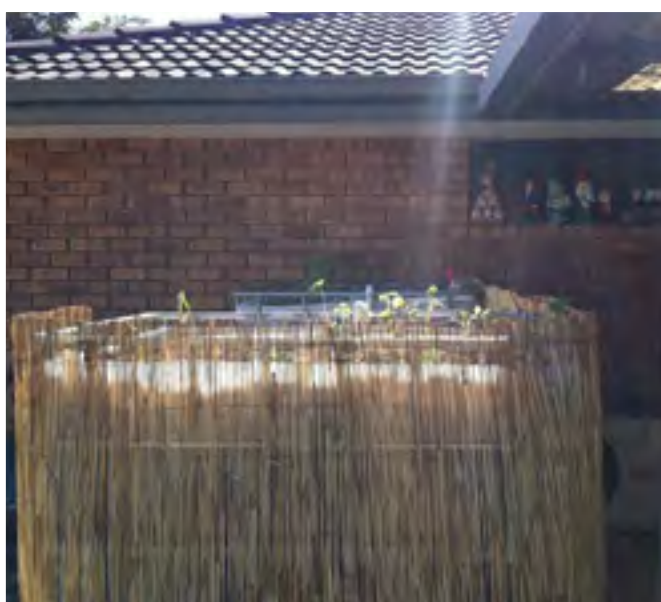
Screens protect the tank from sunlight helping it last longer
