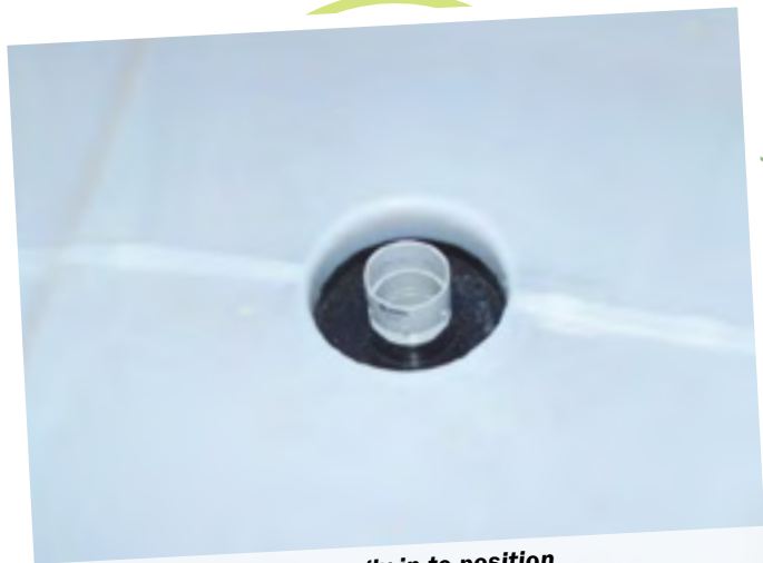
Threaded adaptor fits snugly in to position
