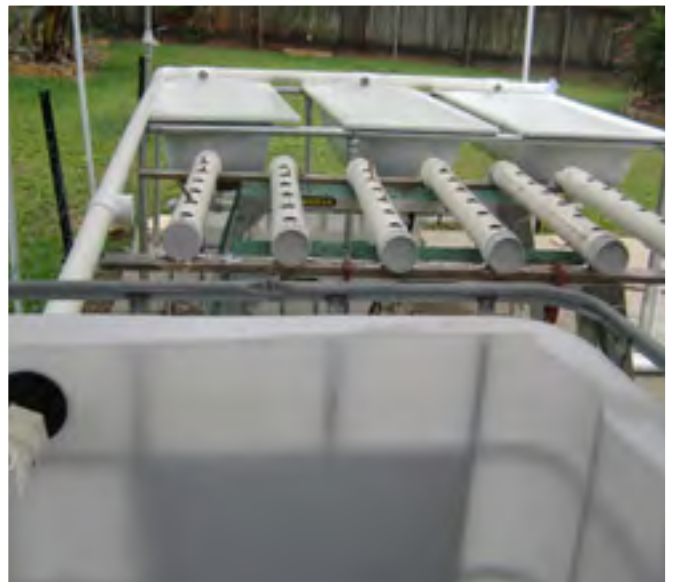
Pipework plumbed and ready to check for leaks
