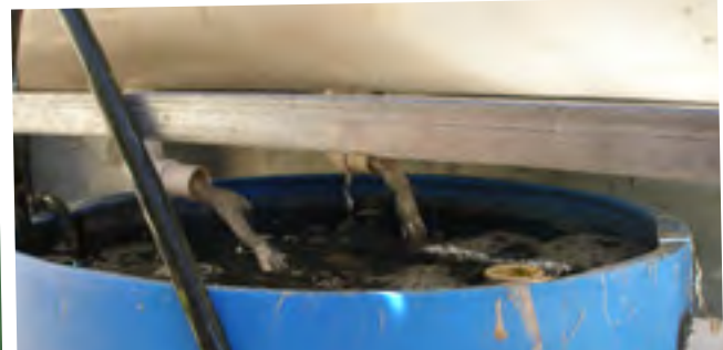
Water is pumped up the black growbed positioned above, returns to the blue barrel as shown here and overflows to the main fish tank.
