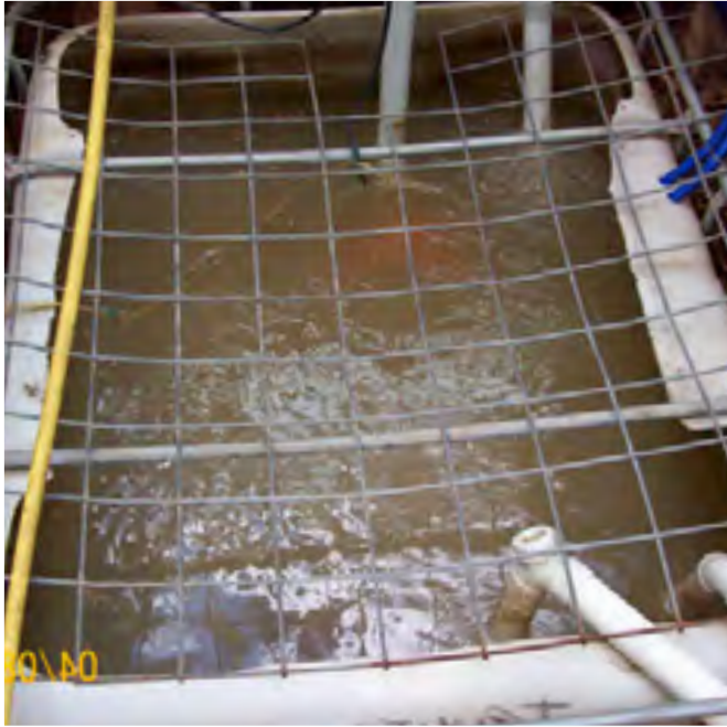
Buried sump tank with air hose dropping down through the lid
