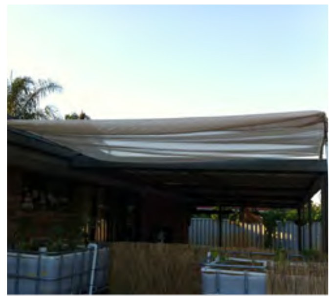
Retractable shadecloth can be pulled across in the hottest part of the day
