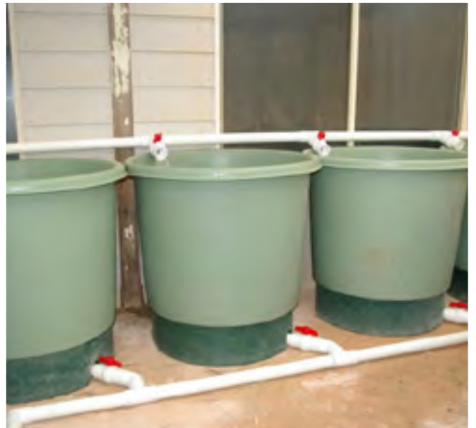
Irrigation and drain lines set out
