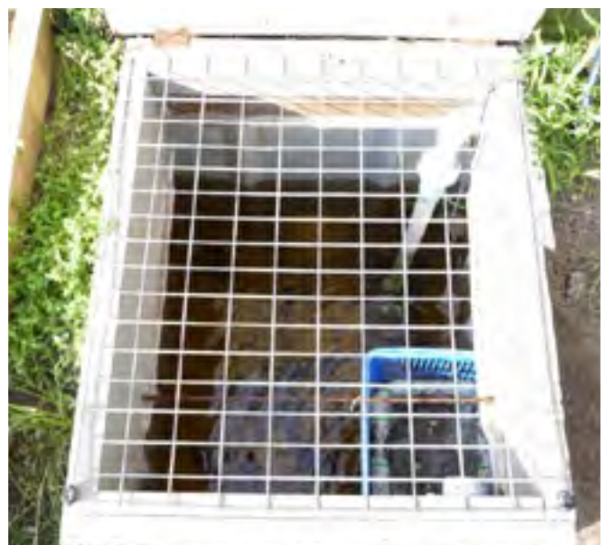
Buried IBC with childproof cover
