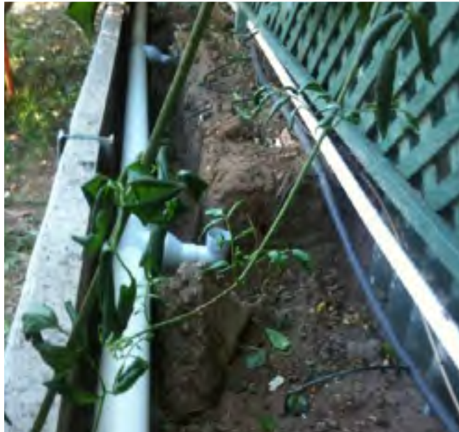
Drain from the barra grow bed ready to be hooked into the new IBC drain
