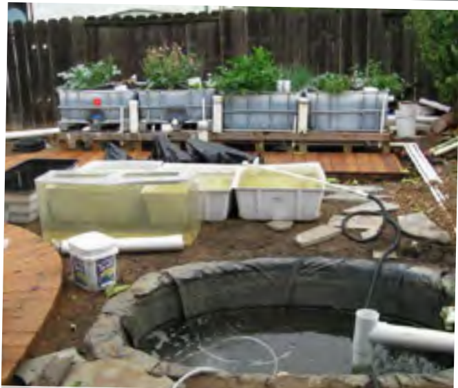
Renovation in progress
