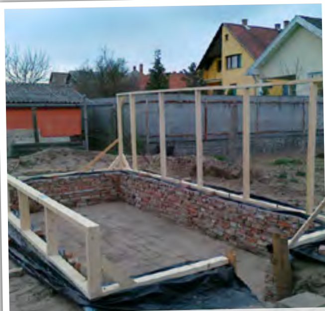
Greenhouse walls being constructed
