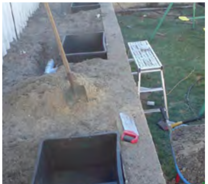
The individual sumptanks for under each bed, buried and plumbed together
