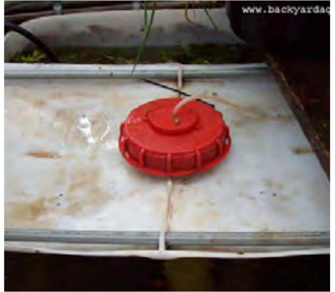
Buried sump tank with air hose dropping down through the lid
