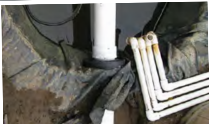
SLO to interconnected ponds and return line from growbeds
