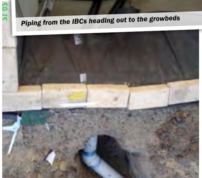
This was a tricky bit of plumbing as the main sump was just a rubber liner
