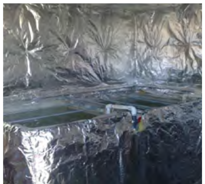
The shed and fish tanks were lined to provide insulation
