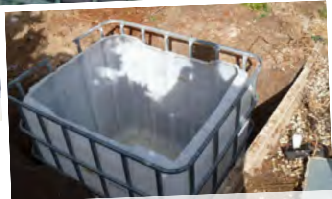
Sump tank finally in it's hole
