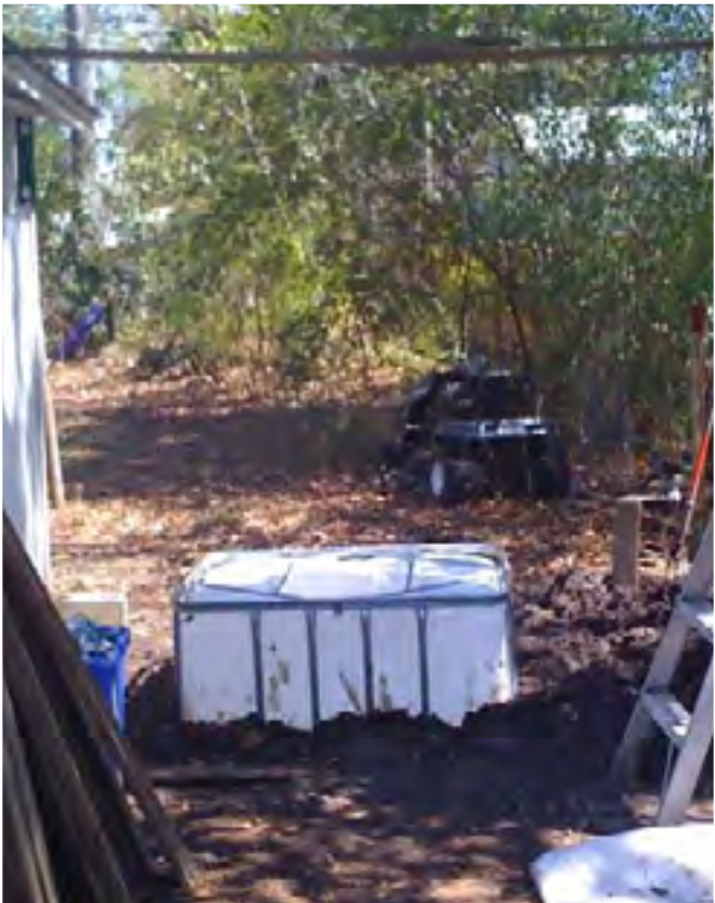
When I was standing waist deep in the hole I was beginning to wonder if I'd lost my mind. The wife questioned my sanity when I was inside the IBC in my swimming trunks with assorted scrub brushes and soaps
