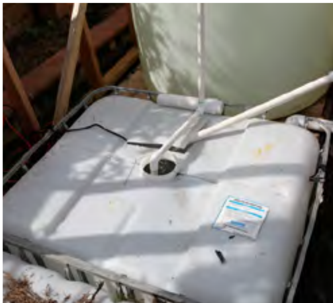
All the growbeds drain into the sump tank before the water is pumped back into the fish tank
