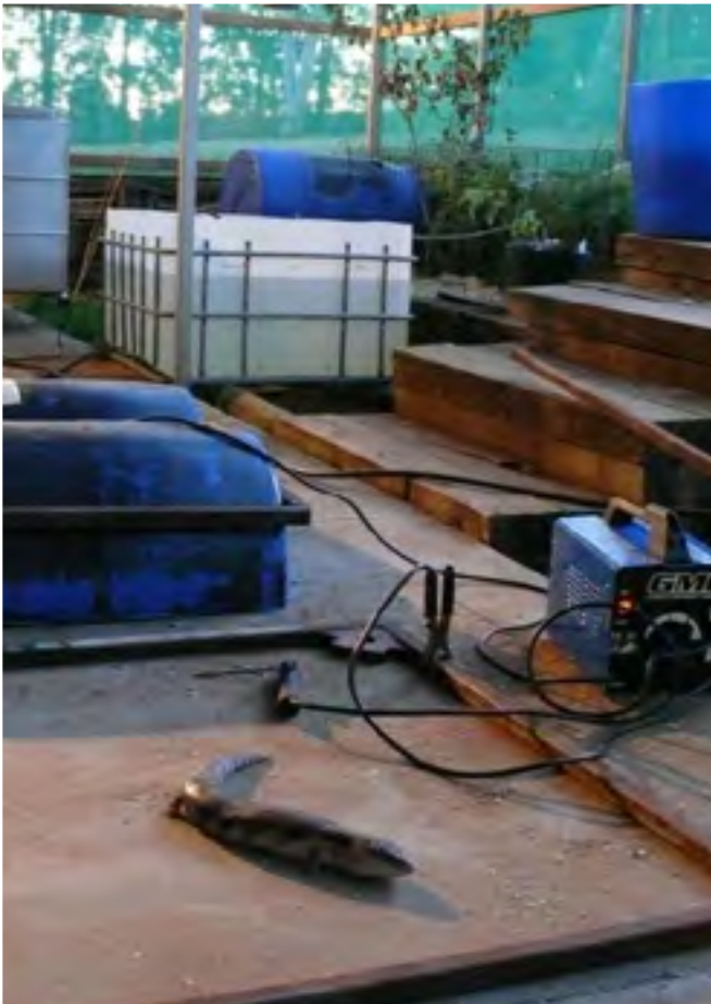
Framework for the barrels under construction
