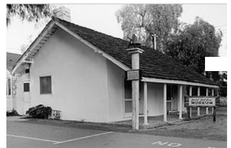
Bancroft House, Spring Valley CA
