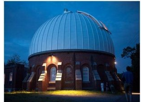
Leander McCormick Observatory at night
