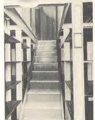
STACK SERVICE STAIRWAY
