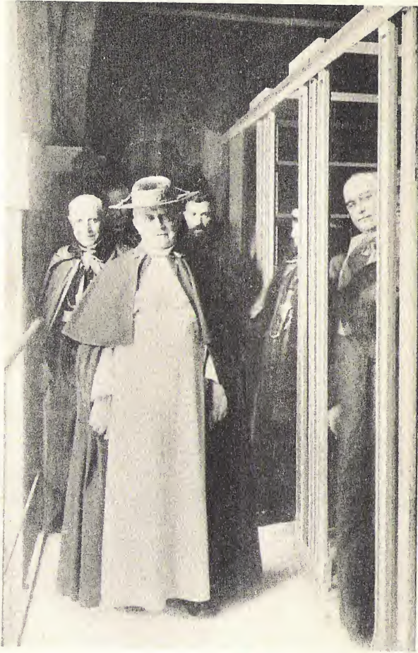
HIS HOLINESS POPE PIUS XI, INSPECTING SNEAD STANDARD BOOK STACK IN VATICAN LIBRARY, DURING CONSTRUCTION
