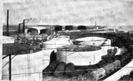
GENERAL VIEW OF SOME OF THE TANKS.
