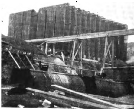
ATMOSPHERIC CONDENSER.
