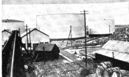
TANKS AND BARRELS.
