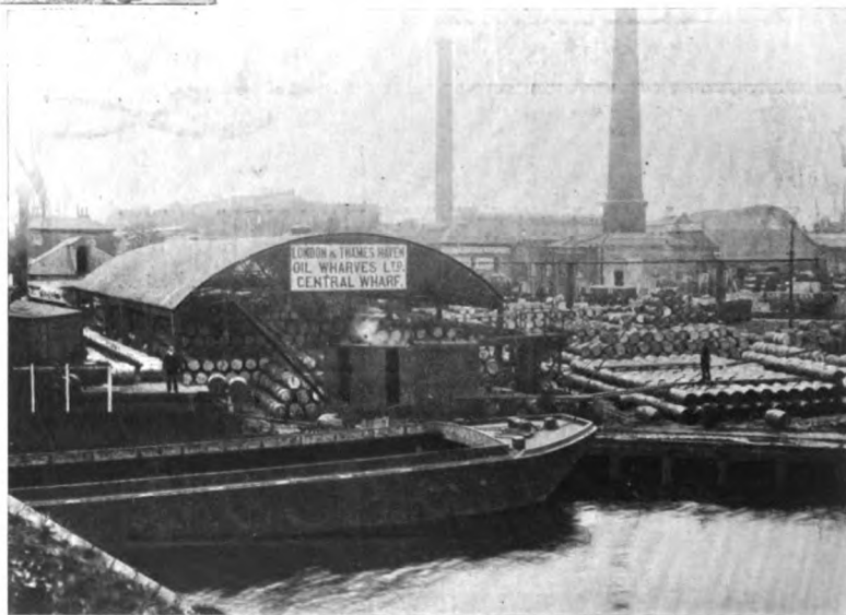
RIVER FRONTAGE AND SHEDS AT CENTRAL WHARF, BOW, LONDON, E.
