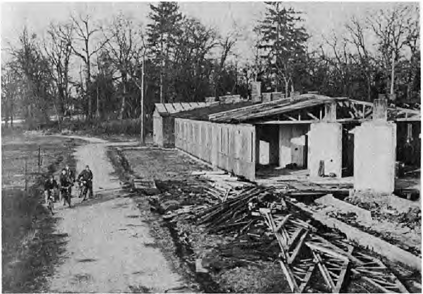
The Biederstein Youth Center in construction
