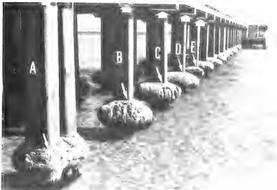
Figure 4. The pier at Dromana, Port Phillip Bay, showing the 'cushions' of Galeolaria caespitosa , exposed at low spring tide on 22 March 1988. Measured on the nearest corners of the concrete supports, the top of the Galeolaria zone (thin arrows) stood 1.99 metres below the horizontal beam (thick arrows) on the double post A, and 1.90 metres, 1.89 metres, 1.86 metres, and 1.90 metres respectively on posts B, C, D and E. Photo: Eric Bird
