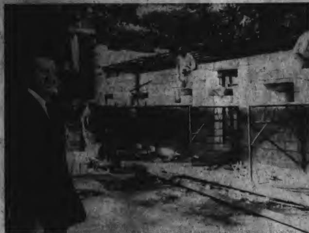
Rev. Hughes watches new construction at Princess Anne Plaza Baptist Church.
