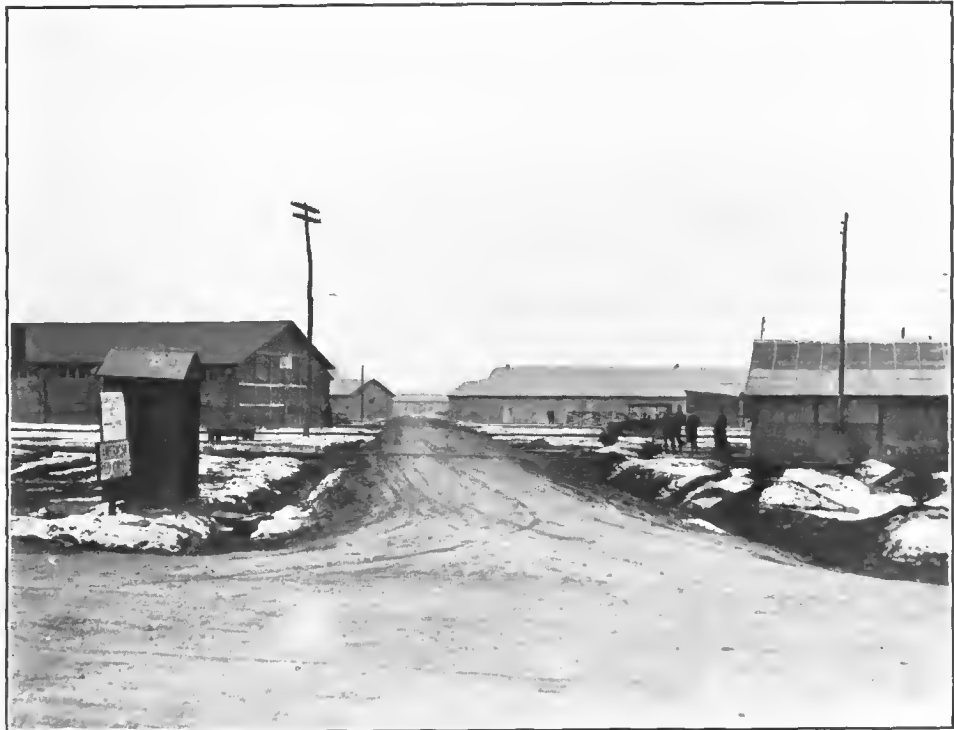
FIG. 43.—Intermediate Medical Supply Depot, No. 2, Gievres; entrance
