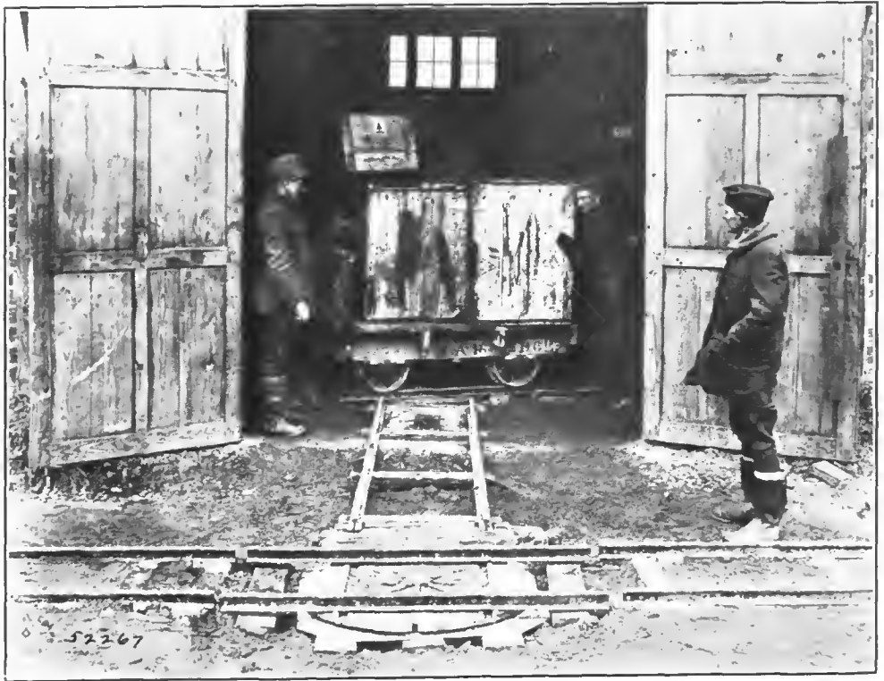
FIG. 48.—Intermediate Medical Supply Depot, No. 2, showing Decauville track and turntable, as used in all warehouses
