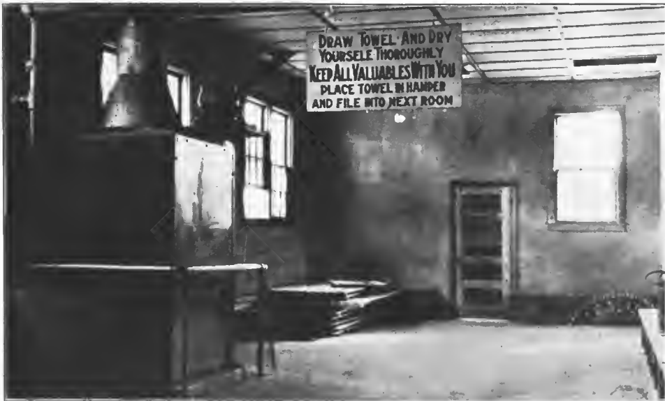
FIG. 88.—Drying room in standard delousing plant, Camp Mills
