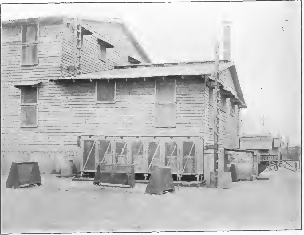
FIG. 54.—Another type of fly-proof shelter for garbage cans outside a company kitchen (located in the ell). Note also the flytraps required by War Department instructions
