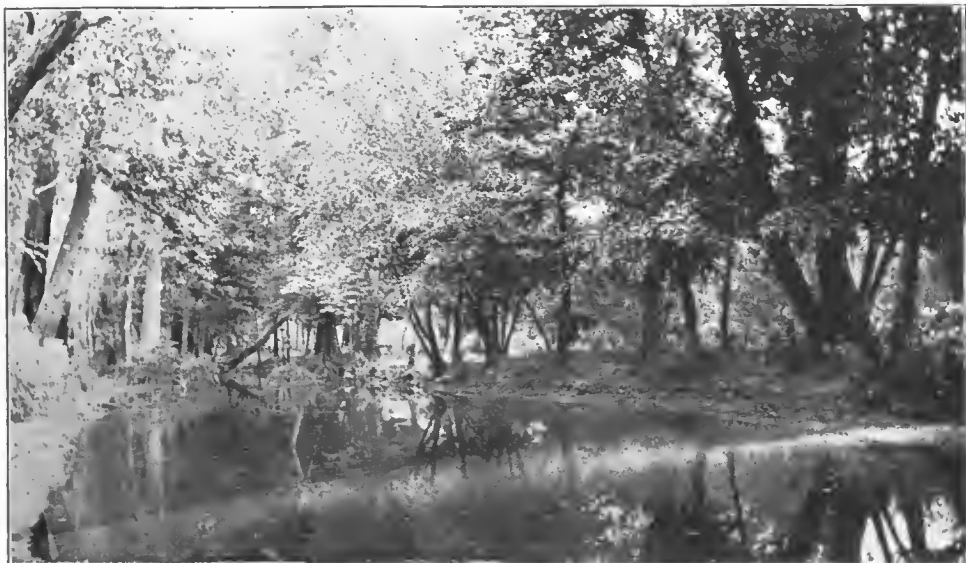
FIG. 68.—Fort Logan II. Roots drainage work; before draining
