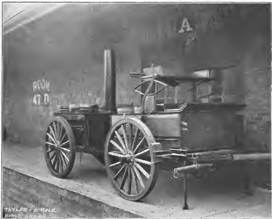
FIG. 45.—The Taylor rolling kitchen No. 30
