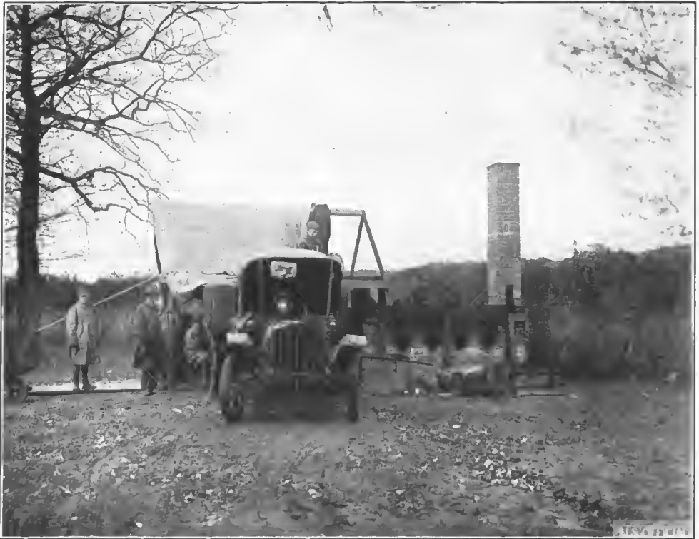
FIG. 108.—Type A incinerator in operation
