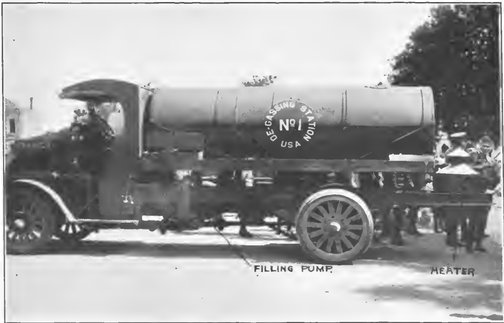
FIG. 119.—Mobile degassing apparatus converted to bathing purposes
