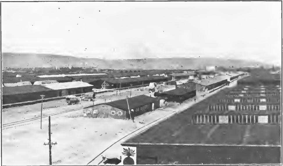
FIG. 143.—Advance Depot No. 1, near Is-sur-Tille, Côte d'Or. On left typical view of warehouse 50 feet wide and varying from 300 to 500 feet in length. By systematic and persistent trapping rats were prevented from becoming unduly numerous here
