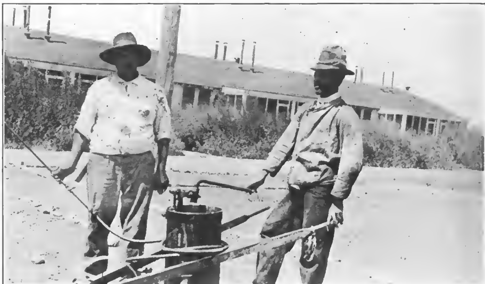
FIG. 63.—Type of oil tank and spray used about buildings of the camp where places to be oiled were readily accessible, Kelly Field, Tex.
