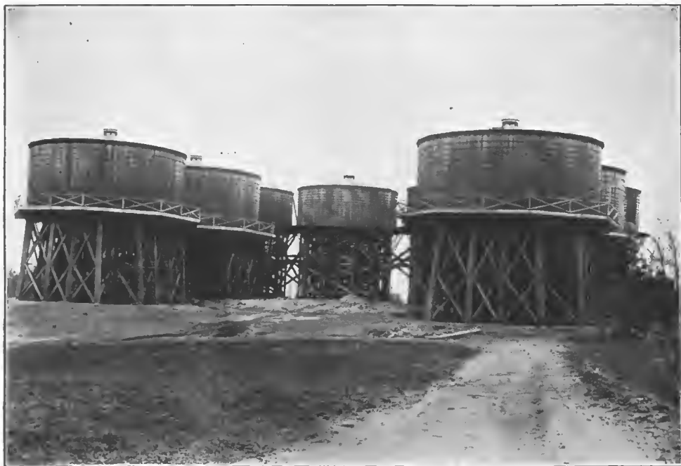
FIG. 35.—Clear-water reservoirs, Camp Meade, Md.
