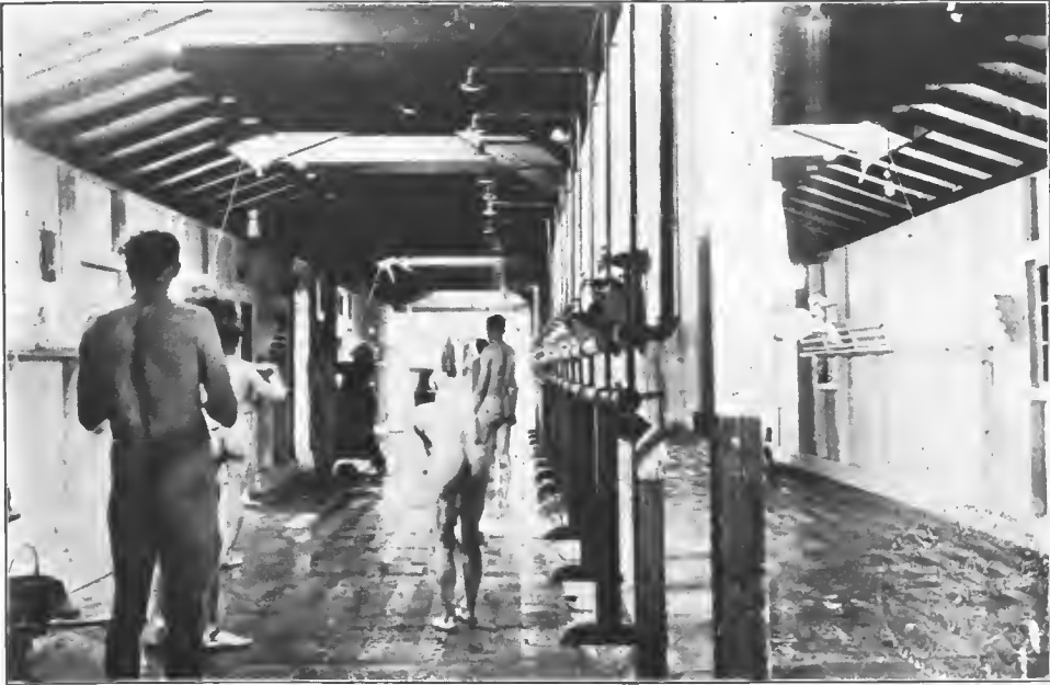
FIG. 87.—Shower room in improvised delousing plant, Camp Mills
