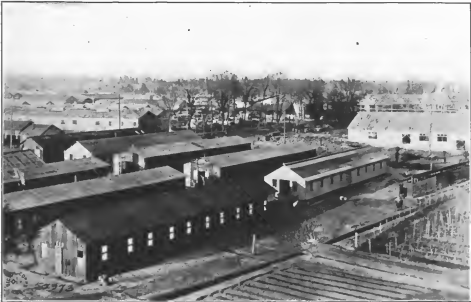
FIG. 9.—Type of troop shelter employed at Camp Génicourt. Note absence of ridge ventilators in buildings in foreground
