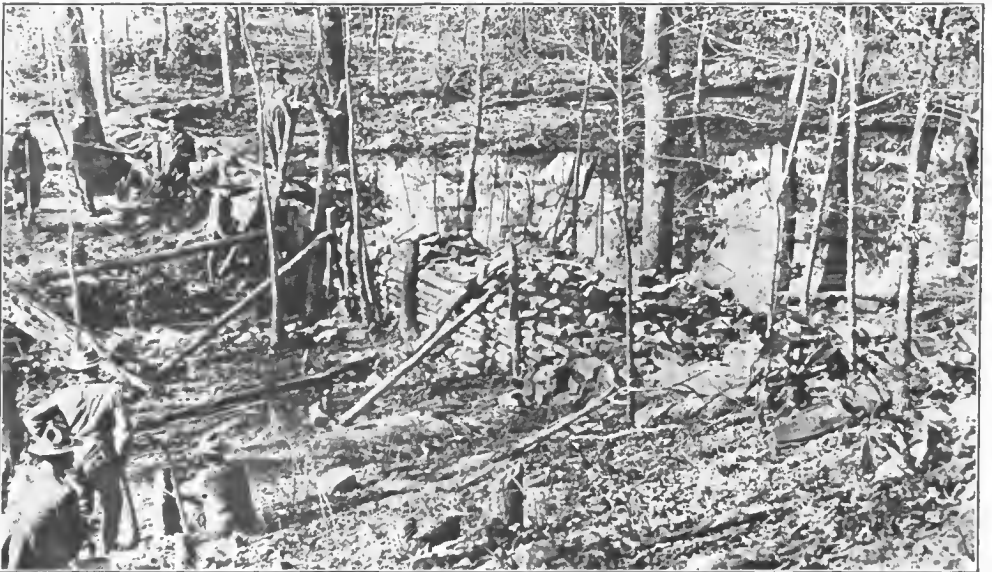
FIG. 72.—Dam for flushing purposes
