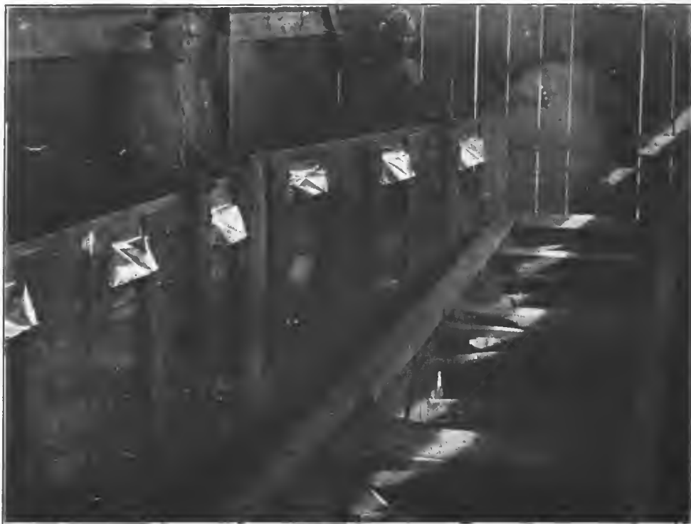
FIG. 85.—Interior of railway latrine, Camp Pontanezen, Brest
