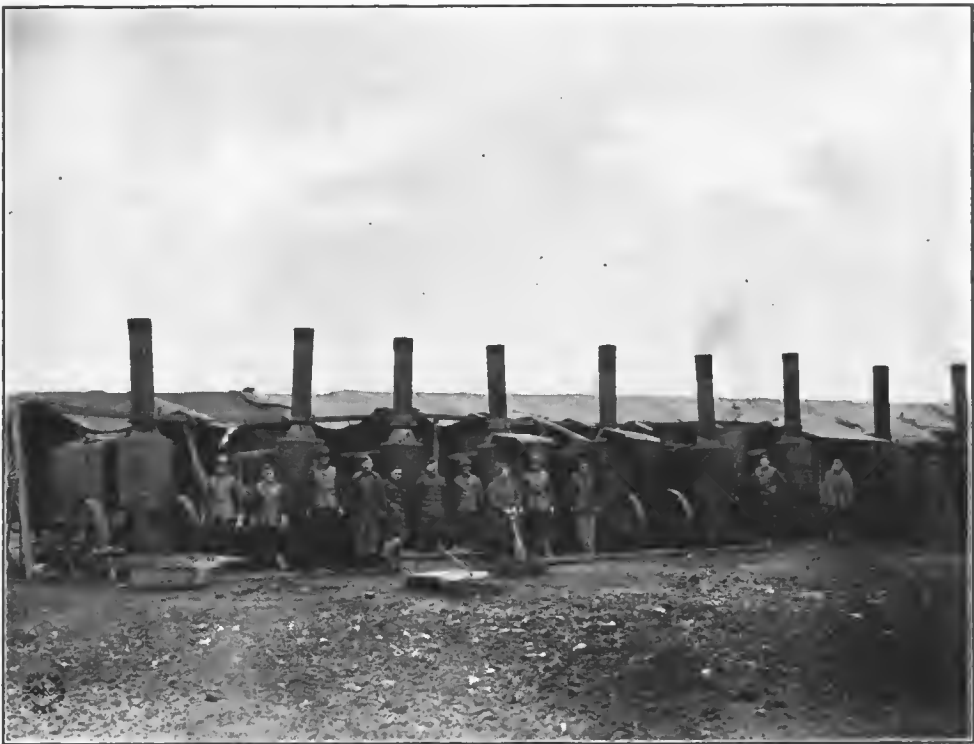
FIG. 126.—A battery of American sterilizers in operation at Camp Hospital No. 11, St. Nazaire
