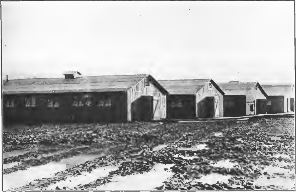
FIG. 8.—Wooden barracks at Camp Ancona, Gironde
