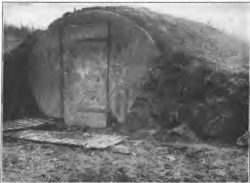
FIG. 138.—German dugout near Damvilliers, Meuse. Note rat holes to the right of the lower edge of door. This type of dugout, with top and sides of heavy corrugated iron, could be made fairly rat proof, but frequently the animals made their entrance through the wooden ends
