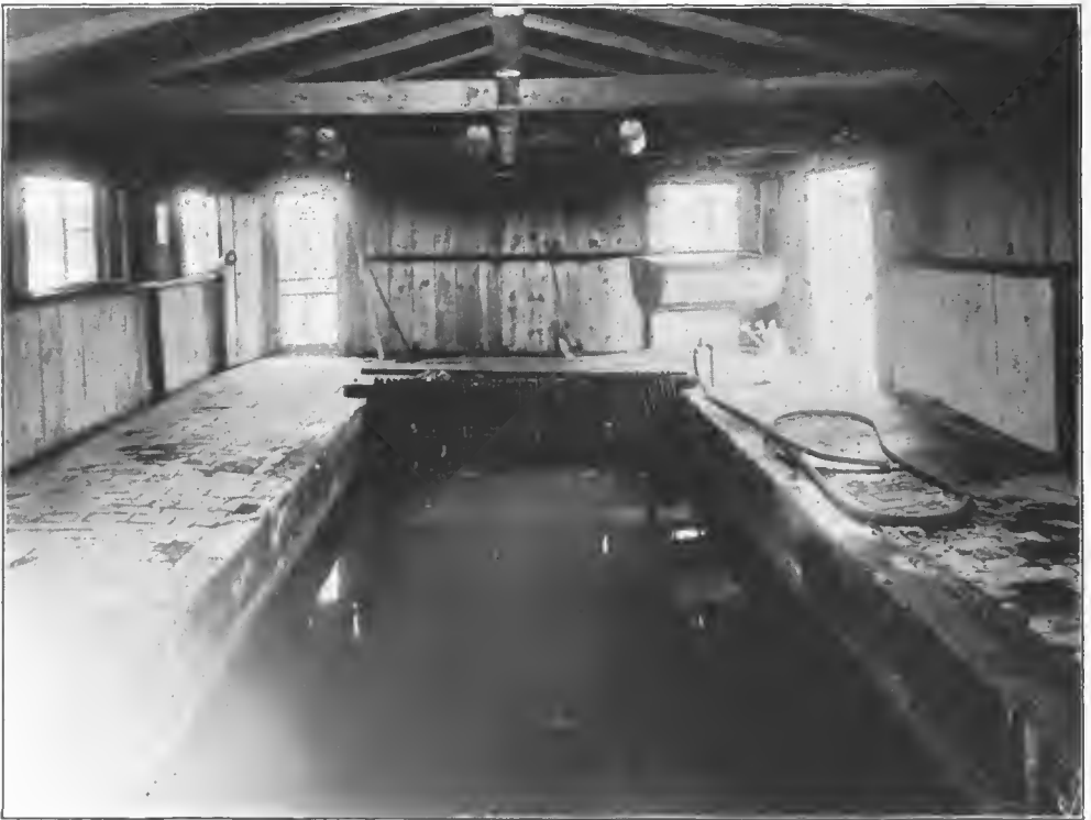
FIG. 42.—Grit and screen chamber, Camp Meade sewage-treatment plant
