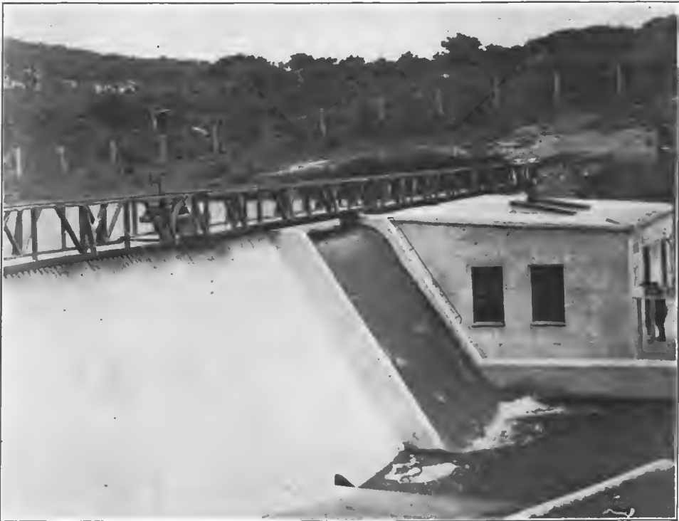
FIG. 52.—Penfield Dam, Base Section No. 5, A. E. F.
