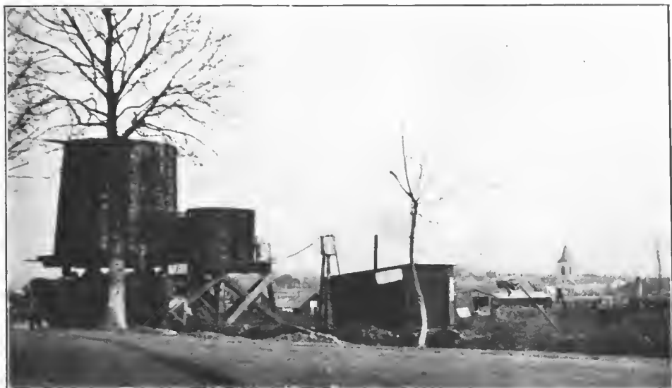
FIG. 55.—Water point, Grosrouvres, A. E. F., showing reservoirs and shower bath
