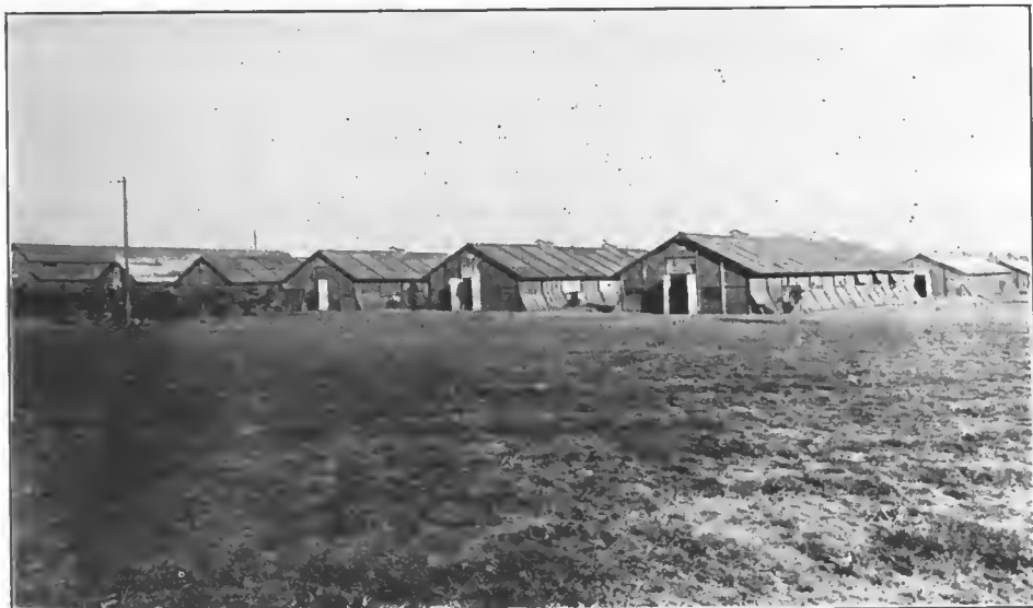
FIG. 3.—General view of old camp at Orange Neuv, Oironde, France, showing Adrian type of barrack
