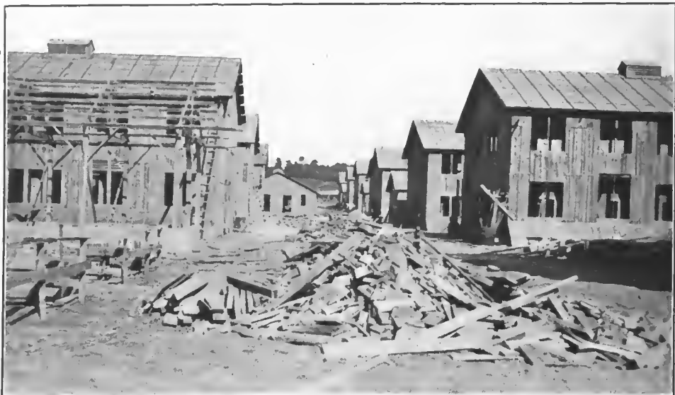
FIG. 6.—Two-story barracks at Camp Baranquine
