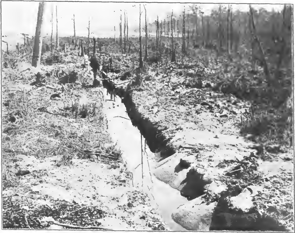
FIG. 71.—Large swampy area, southwest corner Camp Jackson, S. C. This illustrates very clearly the manner in which the ditches are filled with the fine sand after each rain
