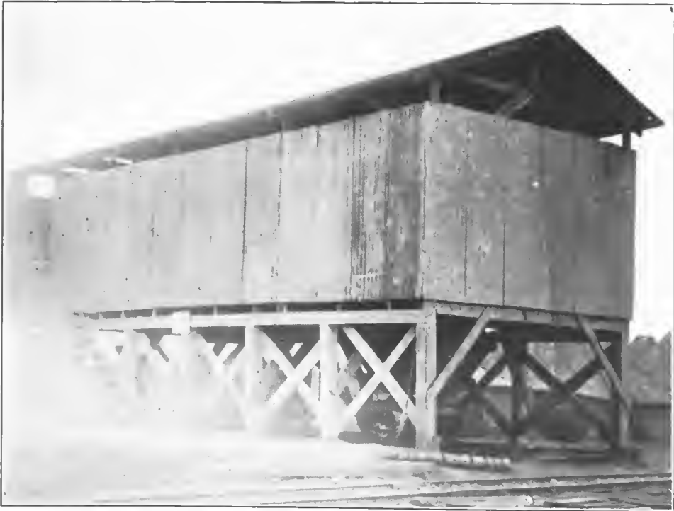
FIG. 84.—Railway-latrine building, Camp Pontanezen, Brest
