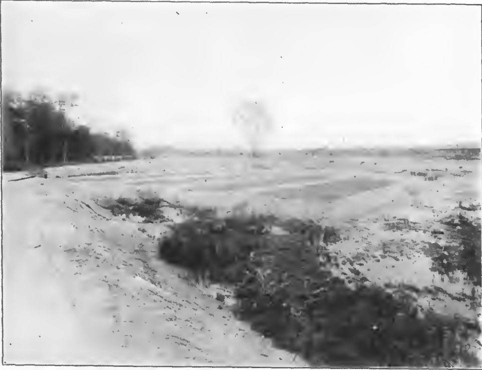
FIG. 43.—Sludge-drying beds, Camp Meade sewage-treatment plant
