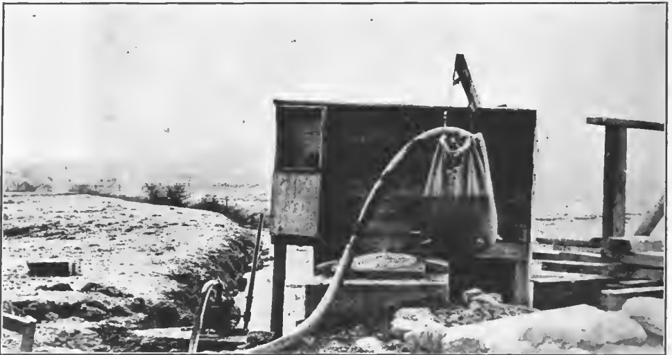
FIG. 64.—Water-sterilizing bag. Typical installation
