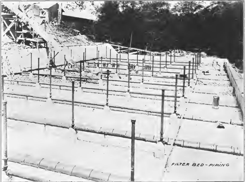
Fig. 44.—Trickling-filter piping before placing crushed rock
