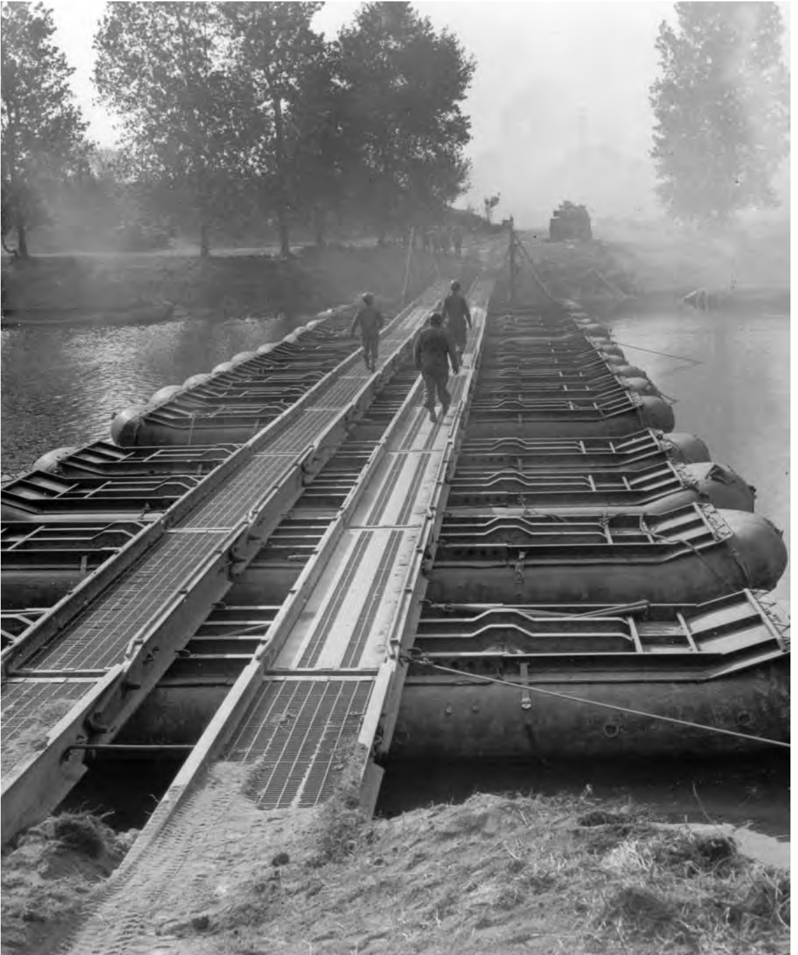
NEWLY CONSTRUCTED TREADWAY PONTON BRIDGE over the Moselle River.
