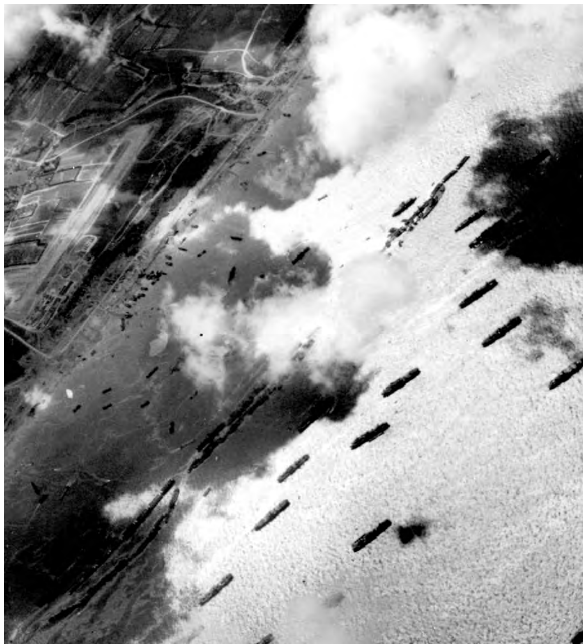
A PORTION OF THE ARTIFICIAL HARBOR AT OMAHA BEACH. This harbor was in the Saint-Laurent-sur-Mer area of Omaha Beach and was known as "MULBERRY A." Breakwaters were formed by sinking ships and concrete caissons, and steel bridging formed causeways to the beach. The harbor, construction on which began on 7 June 1944, was designed to provide moorings for seven Liberty ships and twelve coasters at one time. By 19 June it was 90 percent completed.
