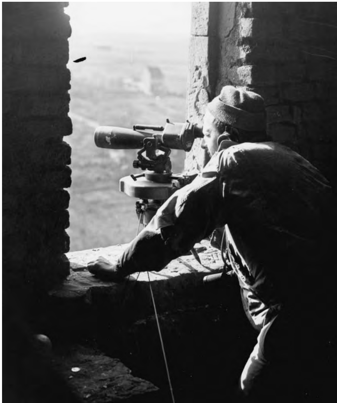
AN ARTILLERYMAN DIRECTS FIRE, using an azimuth instrument M1 for spotting and observing.
