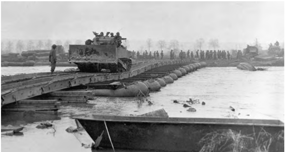
ROER RIVER TREADWAY PONTON BRIDGES. Early on the morning of 23 February the Ninth Army jumped off after a heavy artillery preparation. Covering the right flank was a corps of the First Army. Because the enemy was surprised by this attack only moderate opposition was encountered and by the end of the first day bridgeheads two to four miles deep were held, infantry troops were east of the Roer River, and seven bridges were being completed under a heavy screen of smoke.
