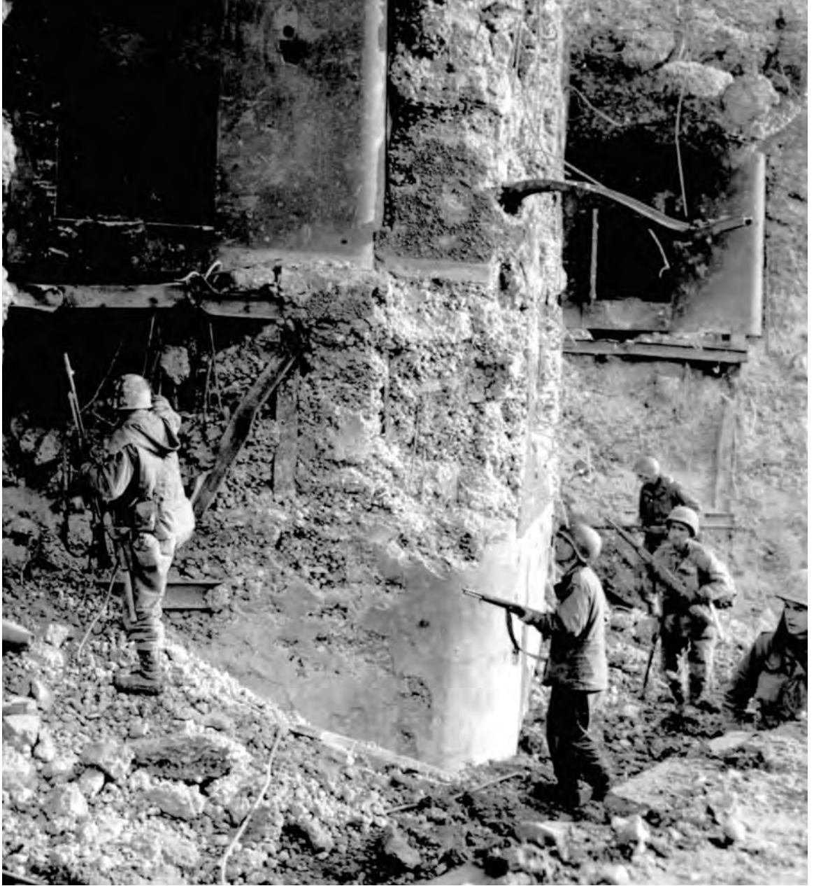
SEVENTH ARMY TROOPS entering a fortress of the Maginot Line, near Bitche, France, which had been taken in the December fighting. Reduction of the strongly defended forts of the Maginot Line was halted when the Arsennes fighting began. The new Seventh Army front included the three following areas: the Saare Valley in Lorraine; the low Vosges mountains; and the northern Alsace plain between the mountains and the Rhine.
