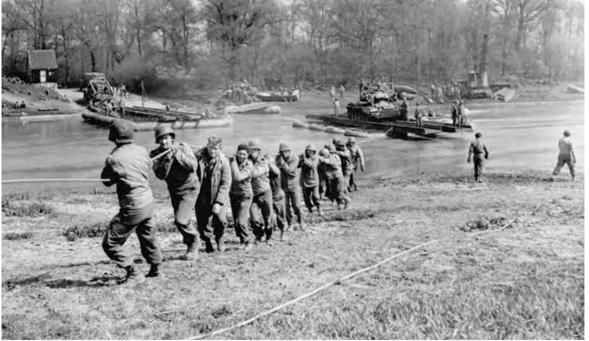
ENGINEERS, building a bridge across the Saale River, pull a tank across on one of the ponton sections (top). Magdeburg, showing the results of bombing (bottom).
