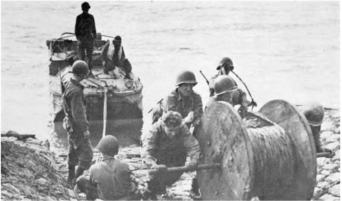
SIGNALMEN ROLL A REEL ASHORE on the east bank of the Rhine after laying a submarine cable on the bottom of the river from a DUKW (top). Destroyed equipment left behind by the retreating enemy (bottom). On 25 March the First Army broke out of their Remagen bridgehead, the Third Army reached the Main River, and contact was made between the British Second Army and the Canadian First Army.
