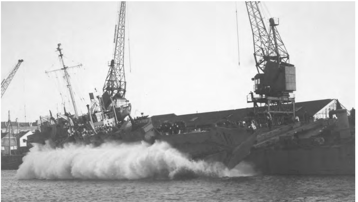
AN LST ARRIVES IN PLYMOUTH, England, carrying an LCT(6) as deckload, after crossing the Atlantic under its own power (top). The LCT was unloaded by sliding it over the side of the LST into the water (bottom). A great many landing craft were needed to mount the coming invasion. These were built in the United States and the United Kingdom.
