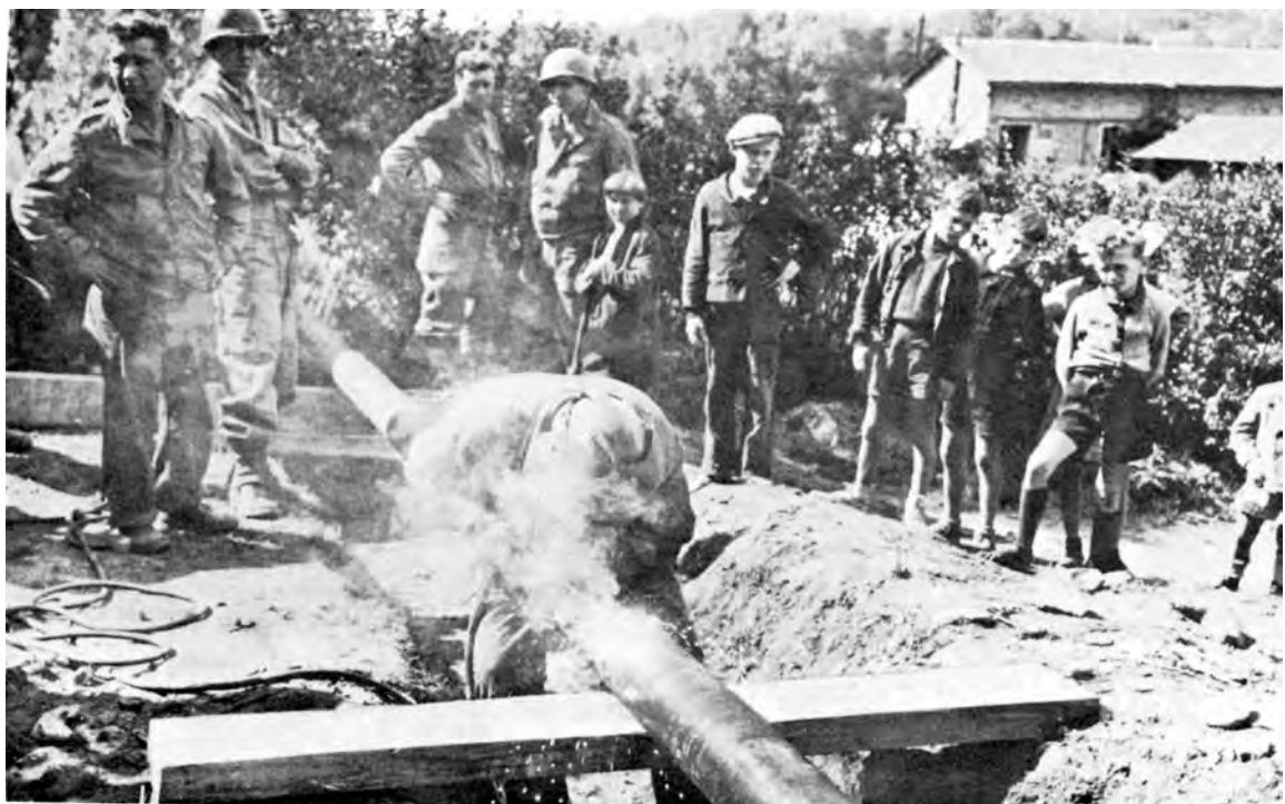
ENGINEERS LAYING A GASOLINE PIPELINE in France. In an effort to transport fuel to the front-line units of the Allies, three fuel pipelines were laid across France. This also relieved the road traffic which became more and more congested as the number of Allied troops in France increased.
