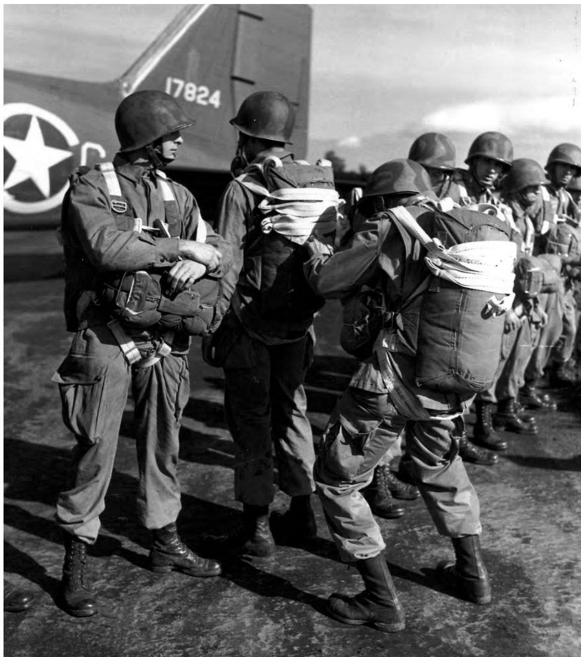
PARATROOPERS having their parachutes inspected before taking off for a practice jump, England, October 1942. These troops were equipped with specially designed clothing and equipment including helmets with a new type fiber liner and chin strap, jump suits with large pockets that could be securely fastened, and boots that laced higher up the leg and which had reinforced toes and stronger ankle supports.
