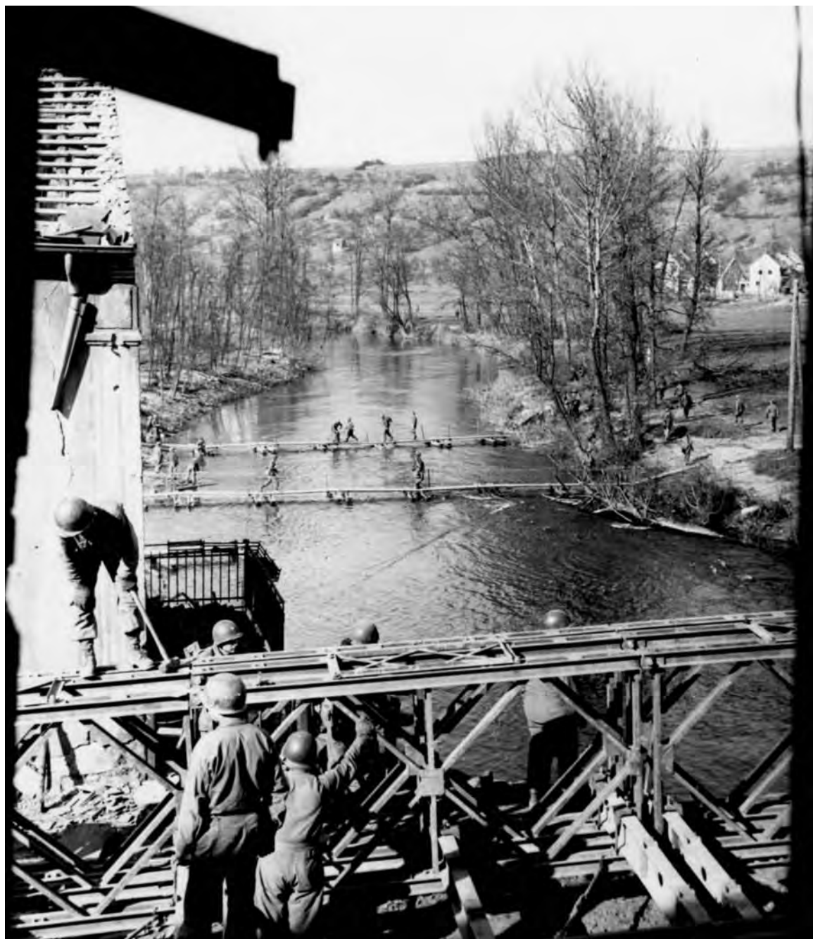
INFANTRYMEN USING FOOTBRIDGES to cross a river while engineers complete a Bailey bridge. On 15 March three corps of the Seventh Army began attacks, one in the heart of the important Saar industrial area around Saarbruecken, the second driving toward Zweibruecken and Bitche, and the third from the Moder River.
