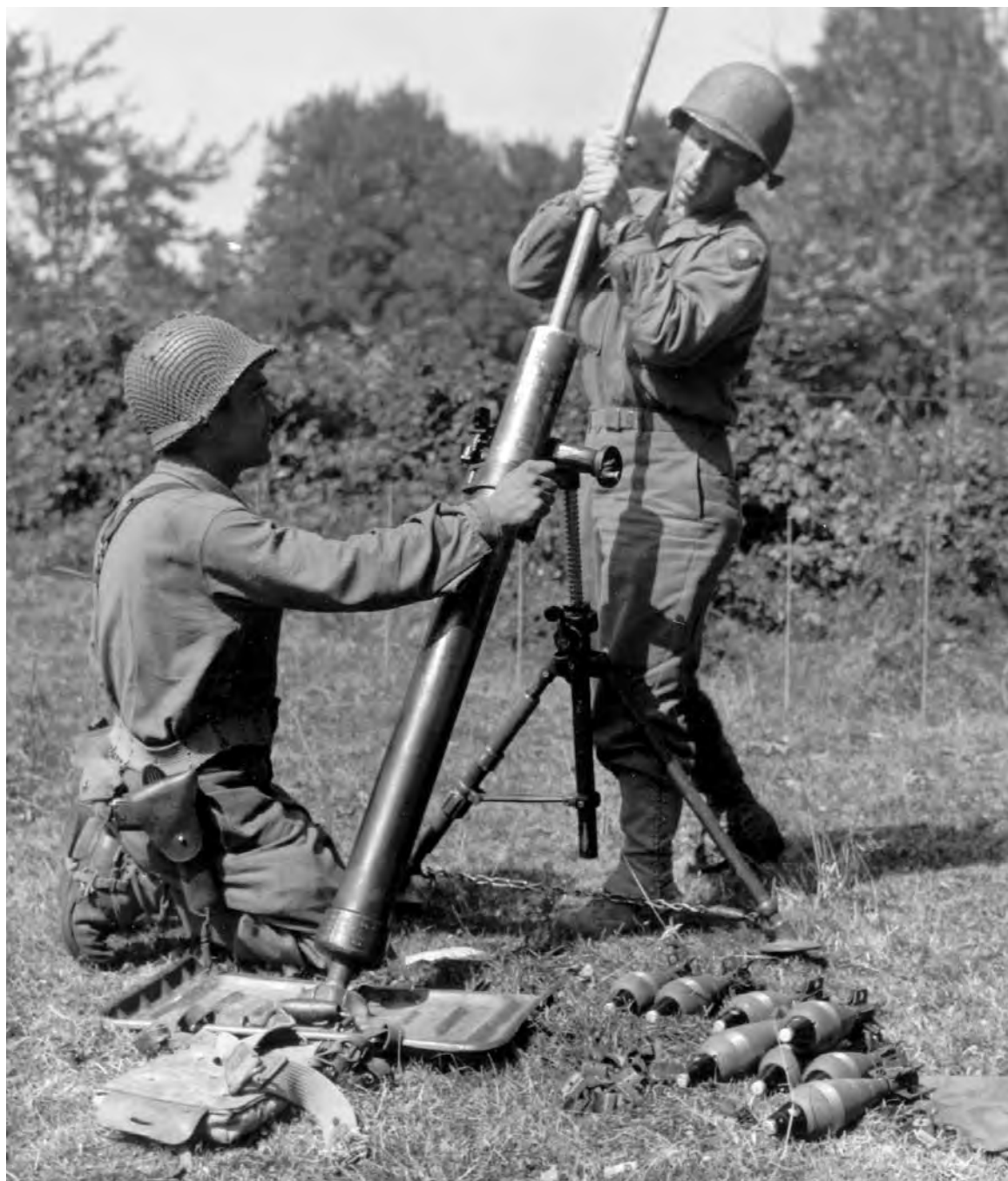
SWABBING OUT THE BARREL OF AN 81-MM. MORTAR M1 before firing. During the battle of the Falaise–Argentan pocket U. S. artillery poured shells of all calibers into the pocket, and Allied aircraft hammered the Germans relentlessly.
