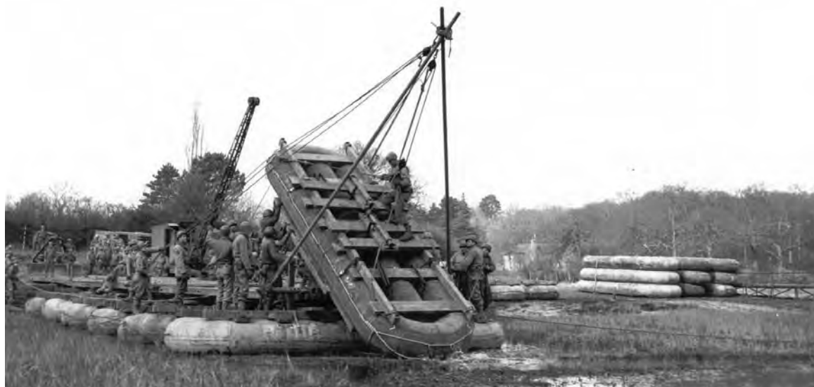
ENGINEERS CONSTRUCTING A PONTON BRIDGE in England during the training period (top). Members of an antiaircraft artillery unit receiving instruction from a British officer while training with a 40-mm. automatic antiaircraft gun M1 (bottom).
