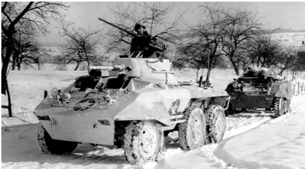
CAMOUFLAGED LIGHT ARMORED GAR M8 and one that has not been painted white, showing the effectiveness of snow camouflaging (top). A crew member of a 90-mm. gun motor carriage M36 throwing paint on the bogie wheels after painting the vehicle (bottom). Tanks, vehicles, and guns were camouflaged with white paint.
