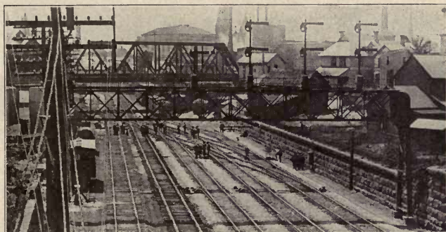
Electrically operated interlocked home signals governing a terminal track arrangement. All signals are indicating "Stop".
