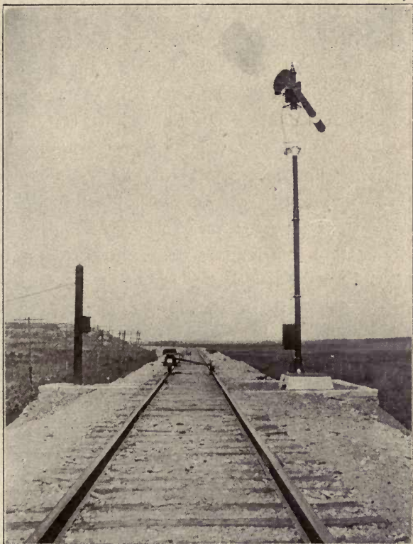
Single blade automatic block signal giving "Clear" indication. This indication is in the lower right hand quadrant.
