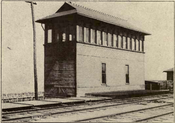
A mechanical interlocking plant, showing lead-out in front of tower.
