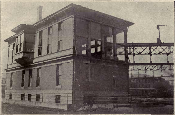
An interlocking tower governing a complicated terminal yard and depot arrangement of tracks.
