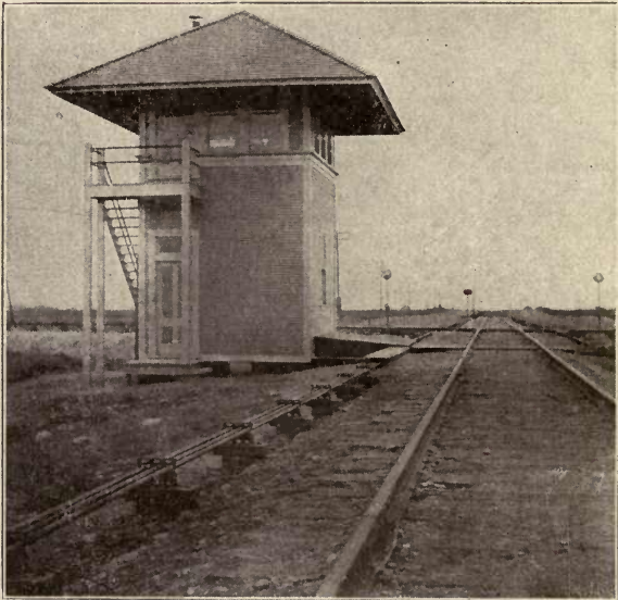
A small interlocking tower. Governs a single track crossing.
