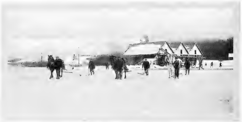
MARKING ICE INTO SQUARES WITH HORSE PLOUGHS.
