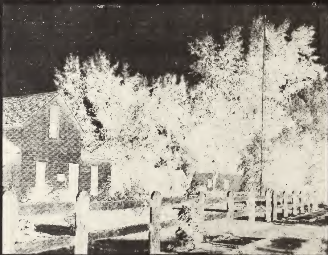
HERE IS THE GRAHAM HOUSE at Blunt that the South Dakota State Historical Society purchased at a tax sale in 1946. The house at that time was dilapidated, without windows and unpainted. The historical group has renovated the house and improved it to the degree noticeable in the above picture. It was in this house that Mentor Graham, "the man who taught Lincoln," died in October of 1885 at the age of 85. The estate is now a shrine to Abraham Lincoln and the man who influenced his life.
