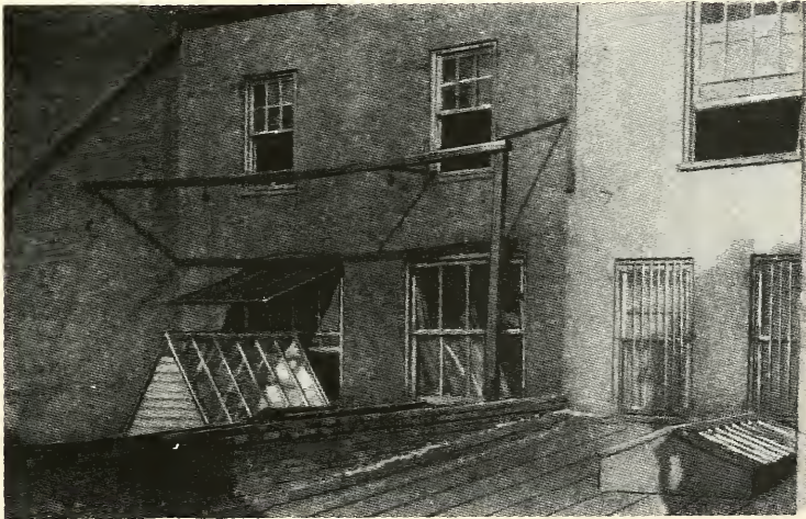
An exterior view of the Lincoln and Herndon law office of 1860. It was upstairs and at back of building. The two large windows on the lower left apparently opened into the office. Here Lincoln formulated many of his political statements. Reproduced from a photograph made in 1886.
