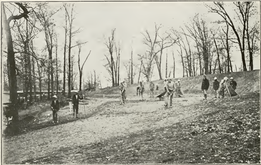
Preparing Site for Lincoln Cabin
