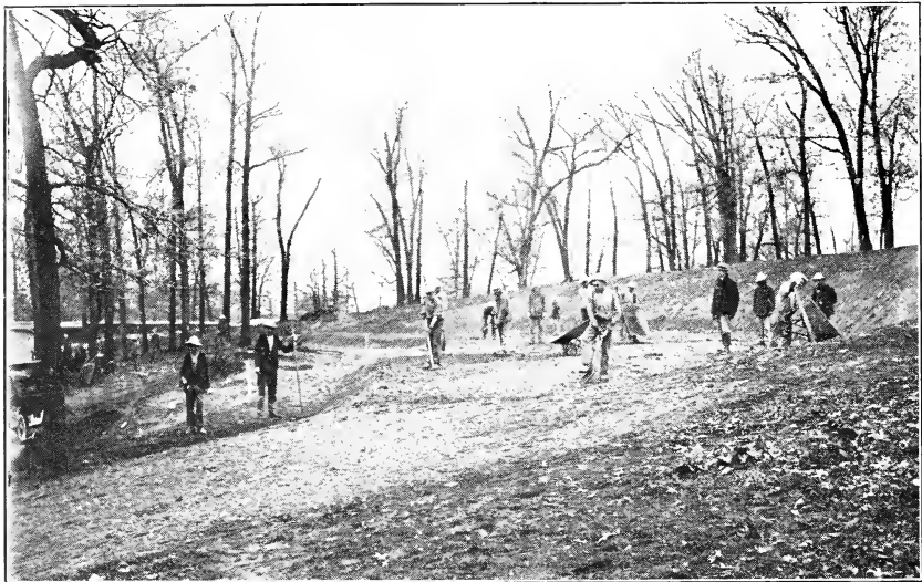
Preparing Site for Lincoln Cabin
