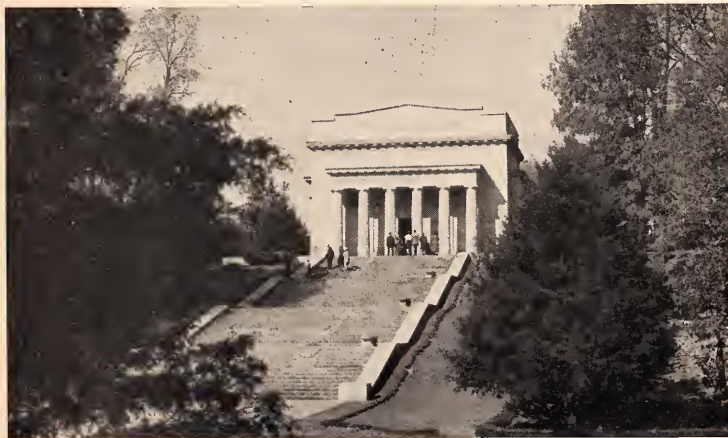
The Memorial Building
