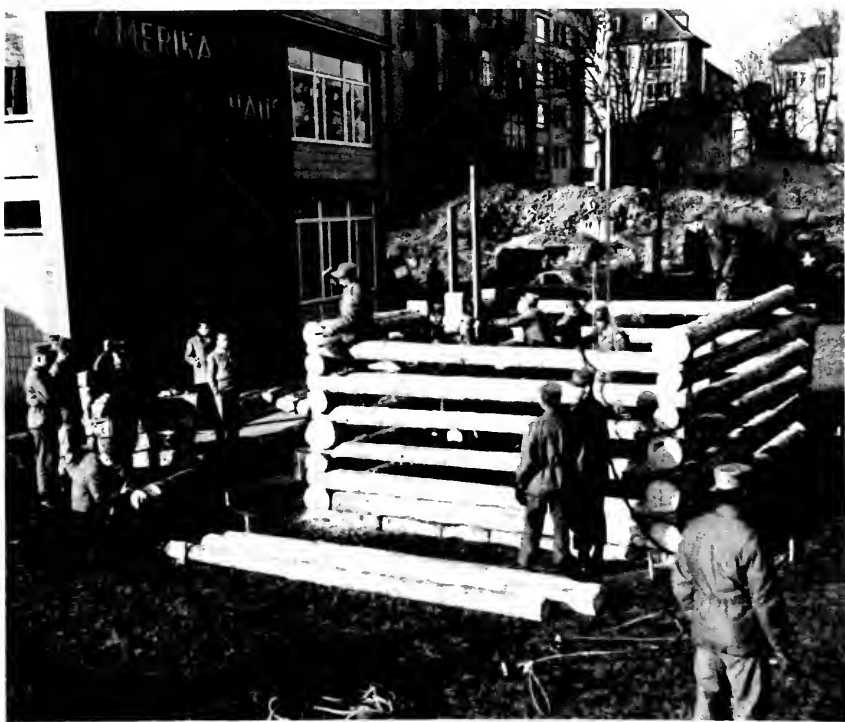
Men of Company C, 299th Engineering Battalion, shown building the replica of Lincoln's birthplace cabin at Frankfurt, Germany.
