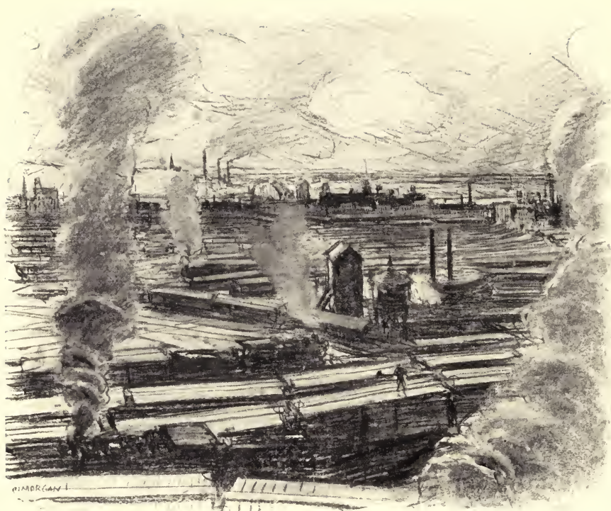
Looking down from Kersey Coates Drive, one sees . . . the appalling web of railroad tracks, crammed with freight cars, which seen through a softening haze of smoke, resemble a relief map—strange, vast, and pictorial
