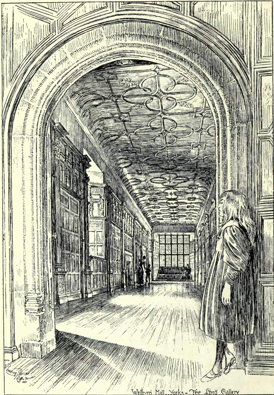
1613. Welburn Hall, Yorkshire, The Long Gallery, WALTER H. BRIERLEY, Architect.
