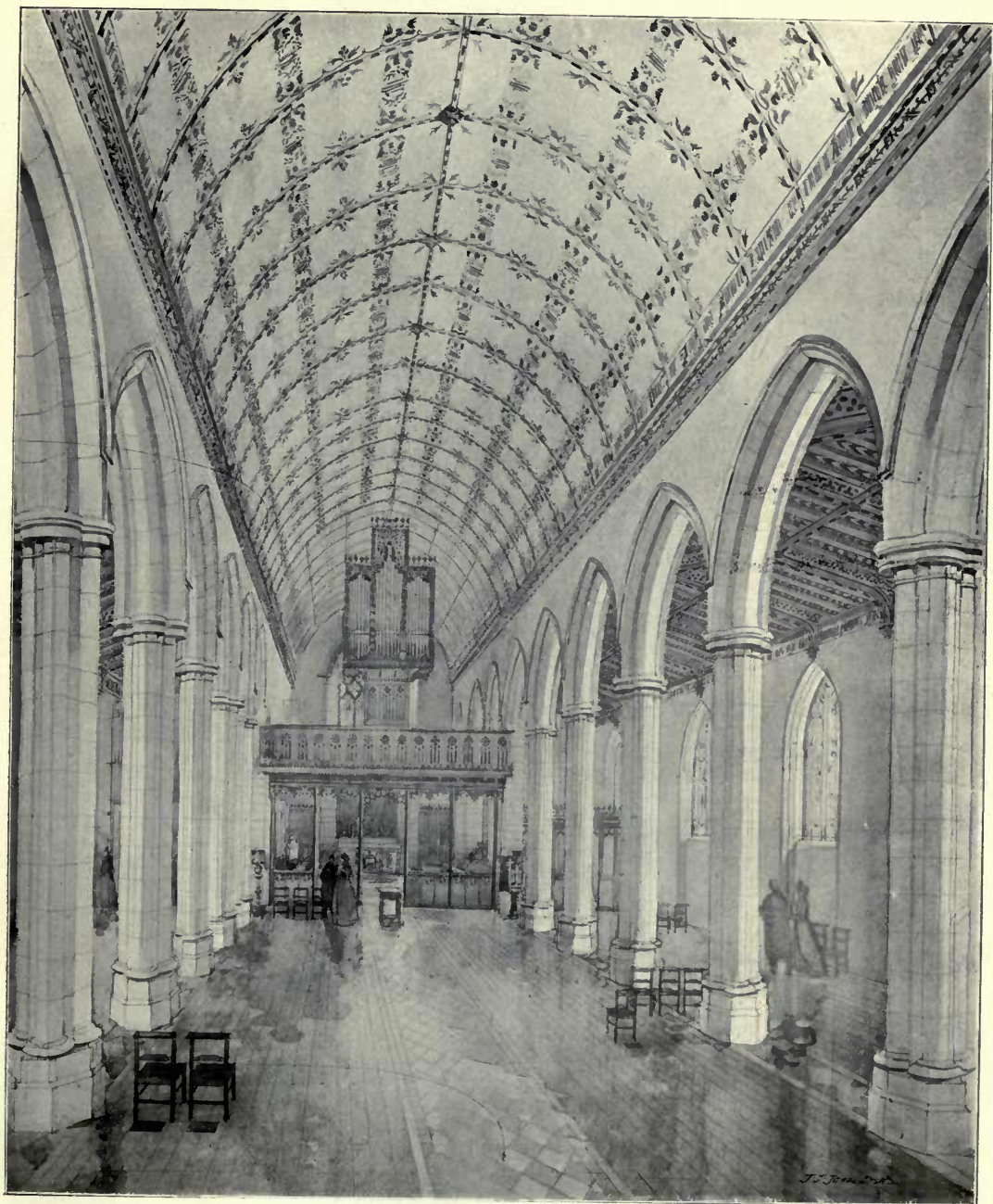
1654. St. Matthew's Church, Chapel Allerton, Leeds , GEORGE F. BODLEY, A.R.A.; Architect. (For Exterior View, see Vol. 14 p 15.)
