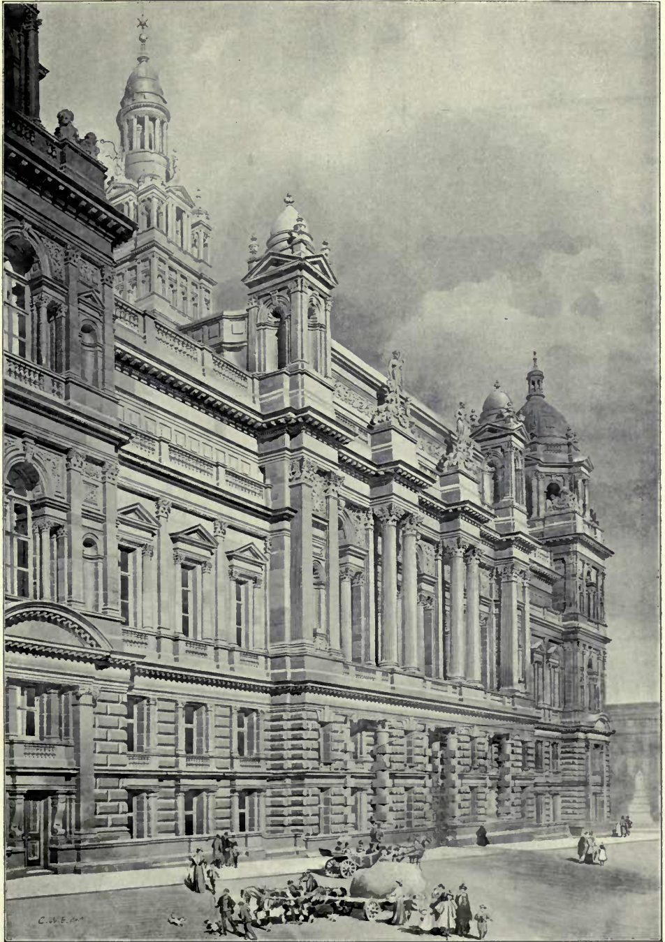
1638. Glasgow Municipal Buildings, John Street Front , THE LATE WILLIAM YOUNG, F.R.I.B.A. Architect.
