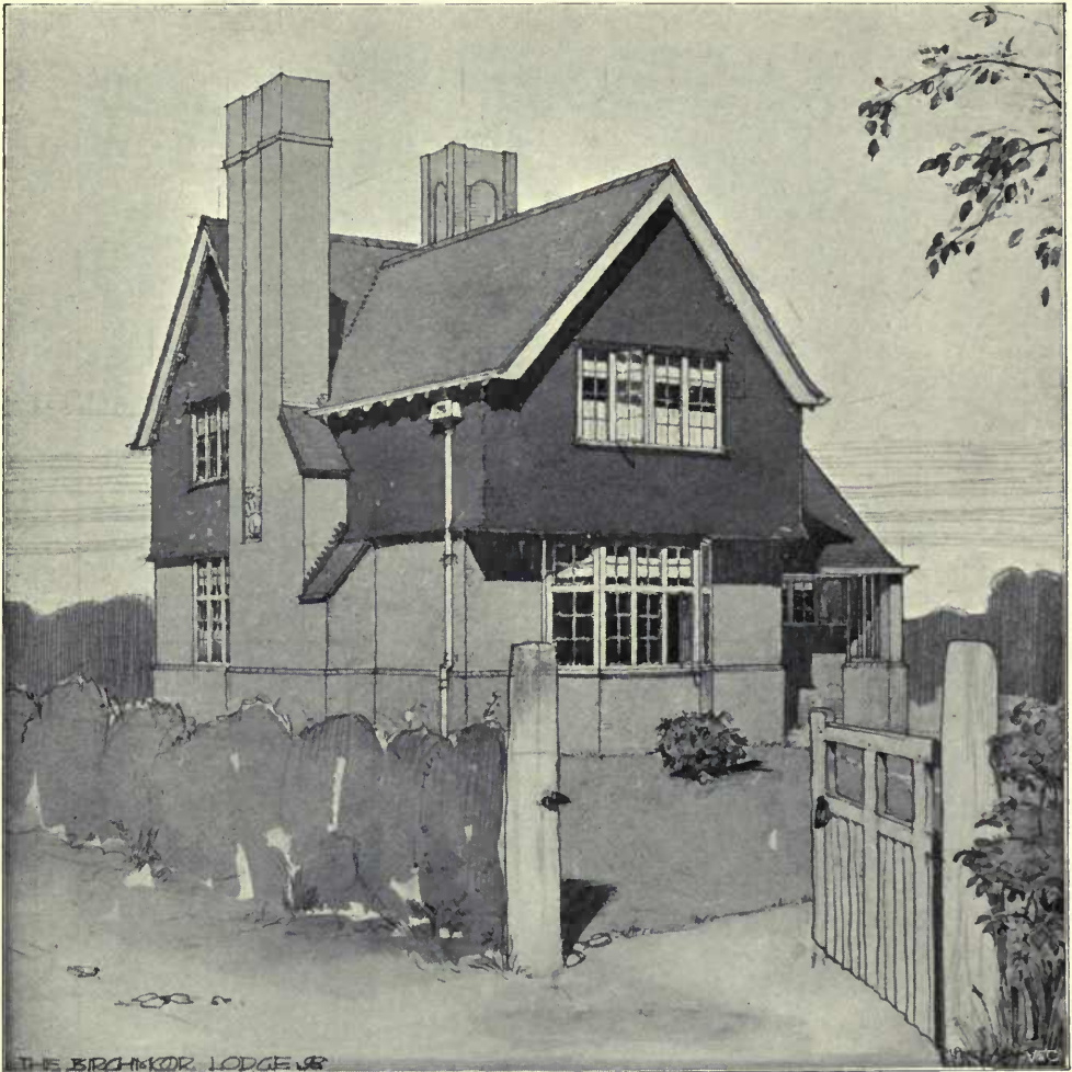
1580. The Birchmoor Lodge, Woburn , H. PERCY ADAMS, F.R.I.B.A., Architect.
