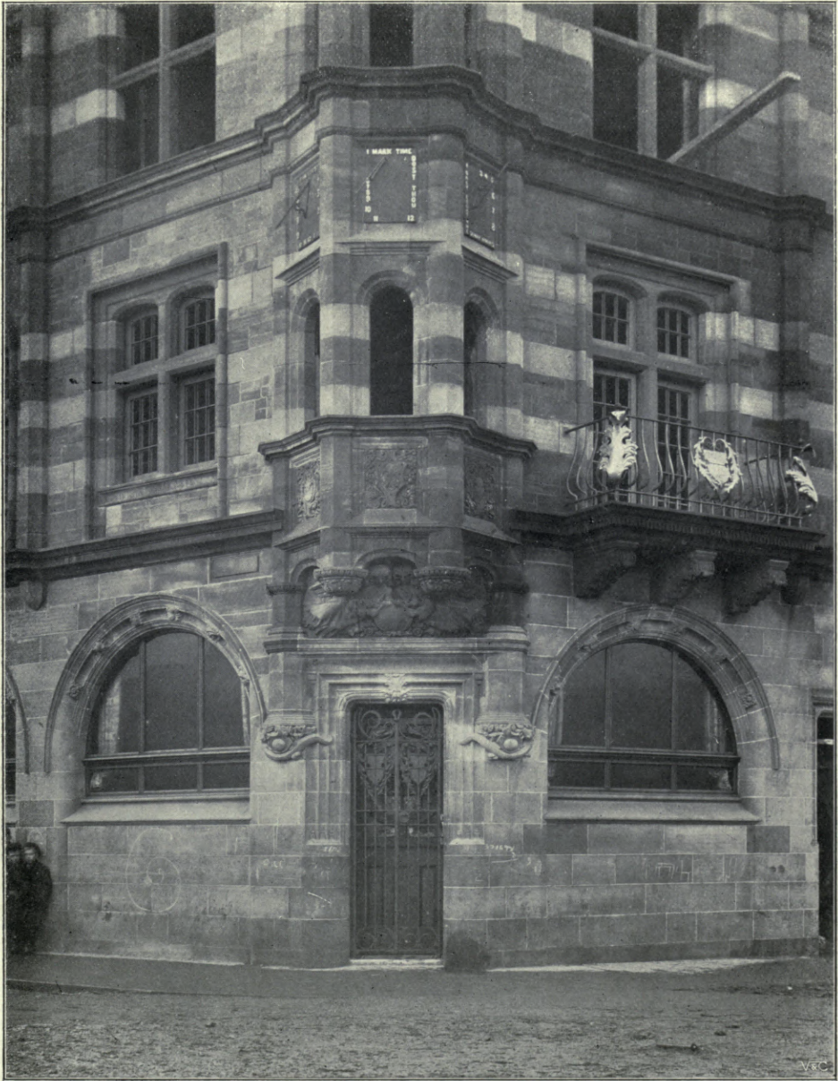
715. Corner Entrance, New Porte Buildings, Burntisland, SWANSTON AND LEGGE, Architects. R.G.I.F.A. Ex., 1901.
