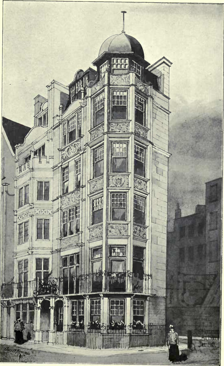
1566. No. 1, Berkeley Square, Mayfair, W., R. GARDNER HAMMOND, Architect. (For Plans, see p. 37.)
