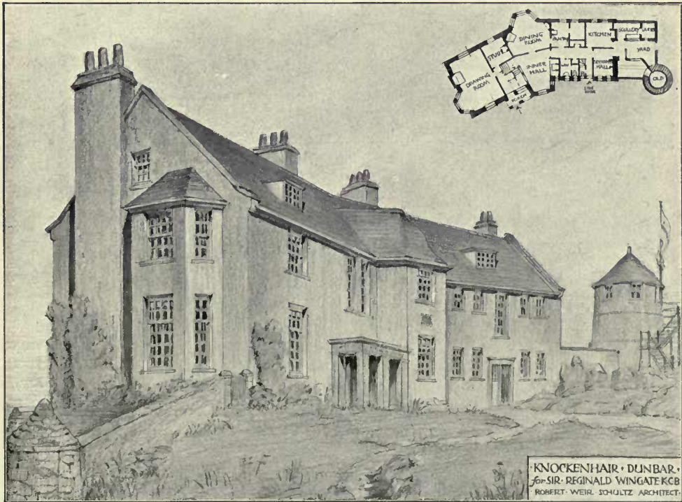
1470. House at Knockenhair, Dunbar, R. WEIR SCHULTZ, Architect. Carpentry and Joinery: R. M'Arthur and Sons, East Linton and Dunbar, N.B.
