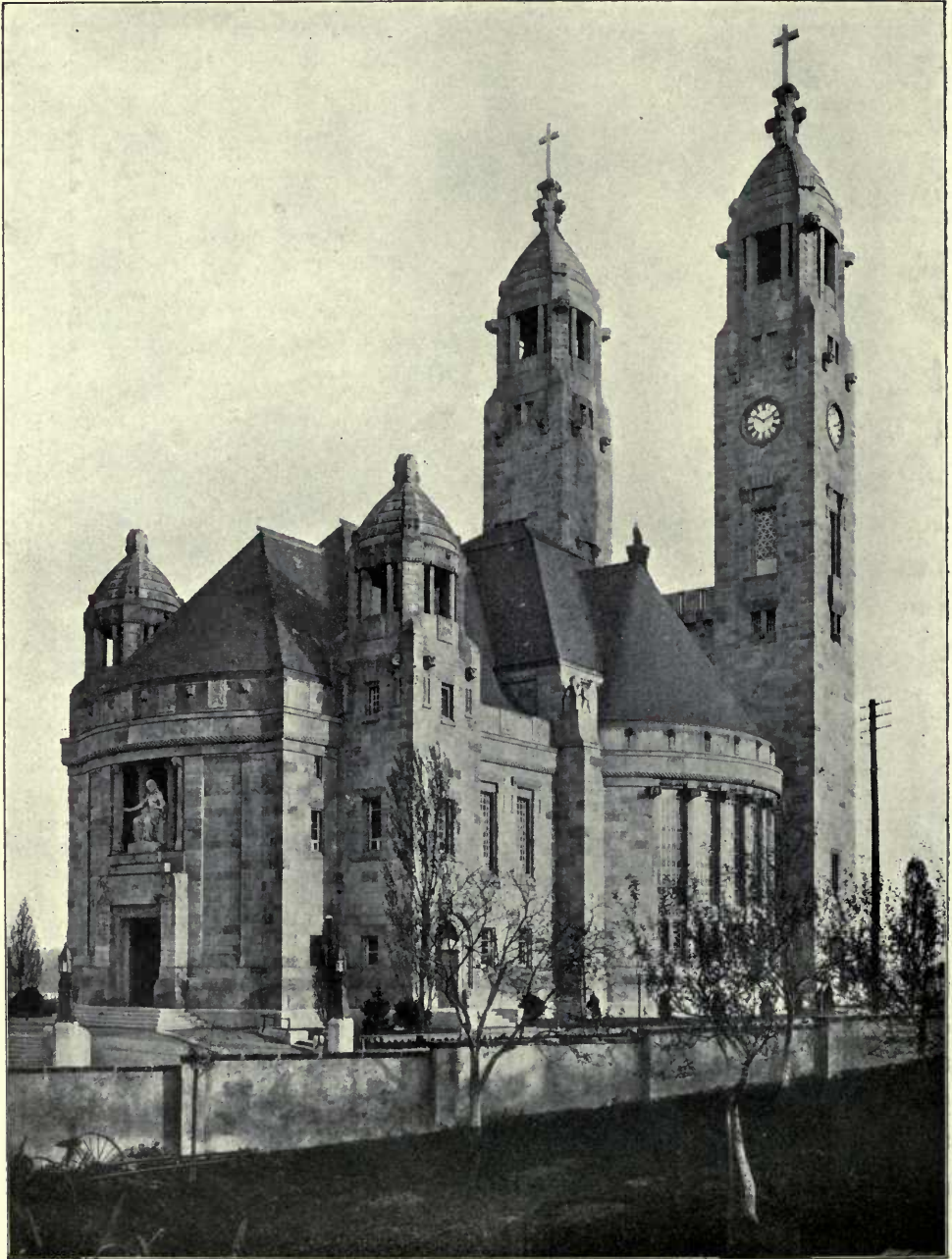
The Protestant Church Strehlen, near Dresden, S.W. View, SCHILLING AND GRAEBNER, Architekten.
