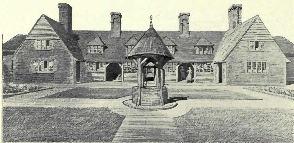
Cottages at Bourne Orchard, Hertford, C. E. MALLOWS, Architect.
