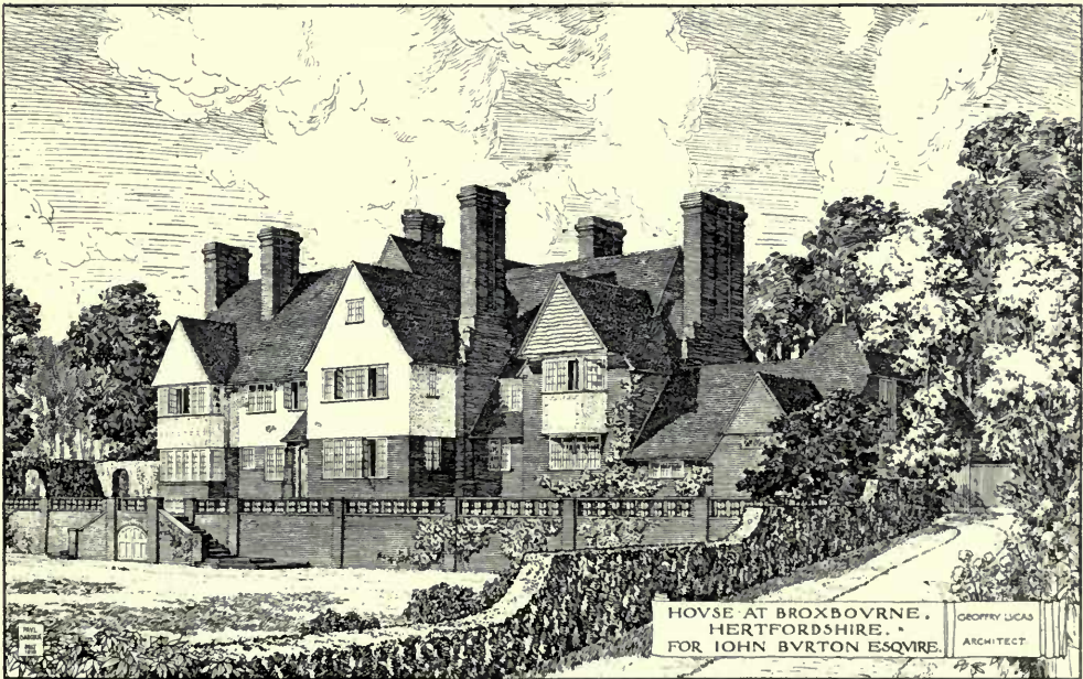
House at Broxbourne, Herts, GEOFFREY LUCAS, Architect.
