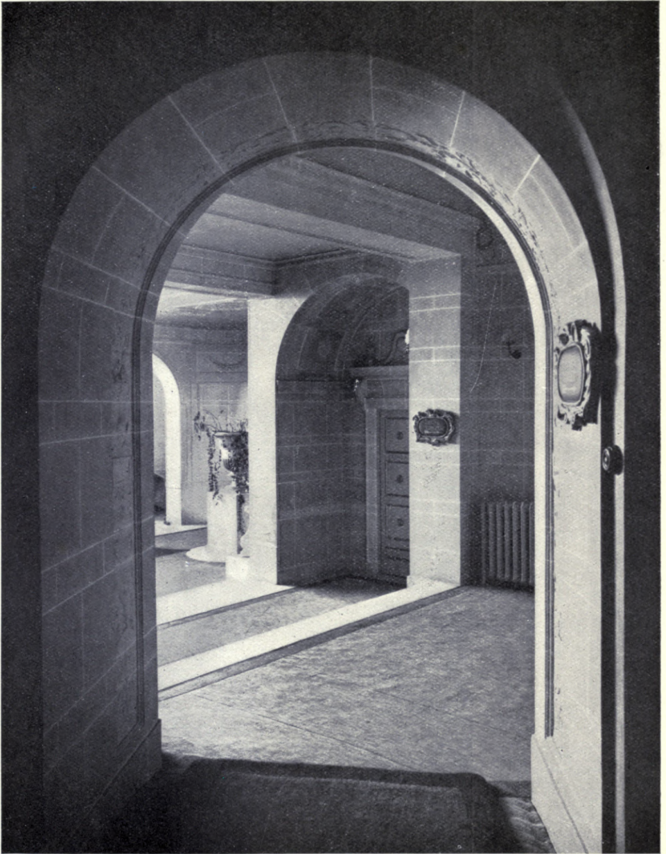
View of Main Entrance Vestibule from Tea Lounge.
