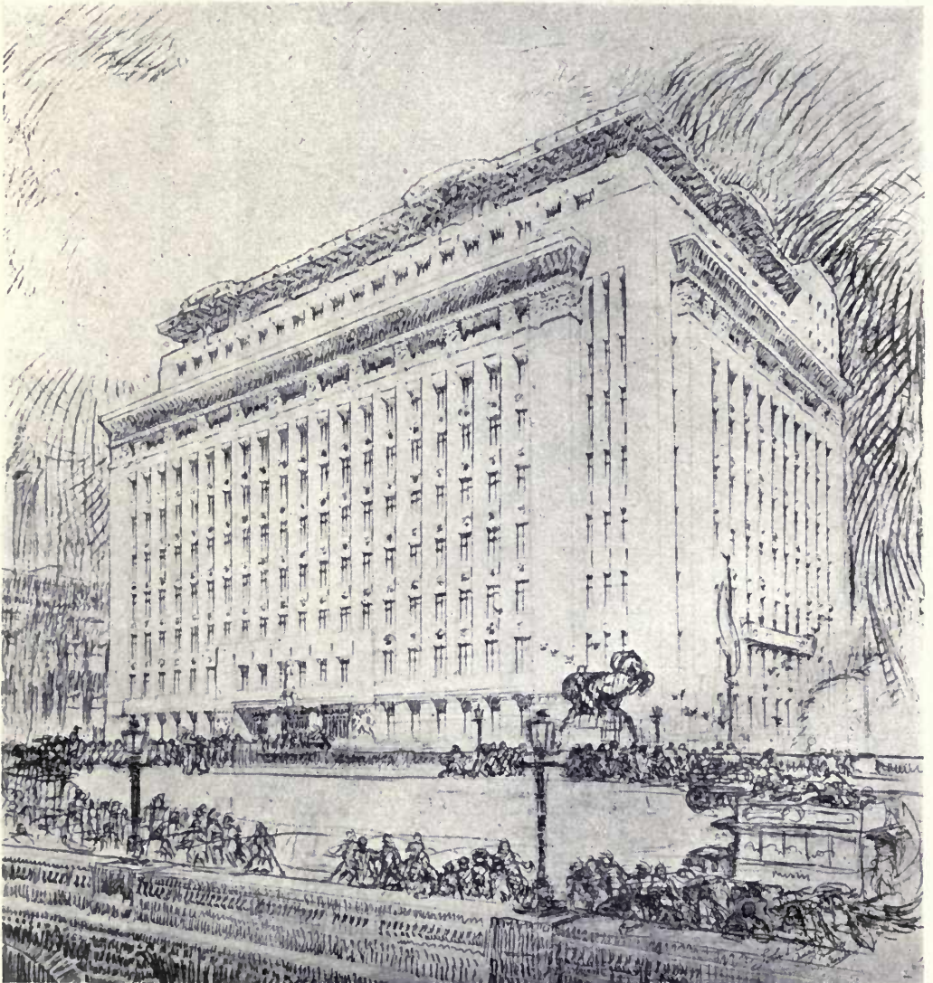
Adelaide House: View from London Bridge.
