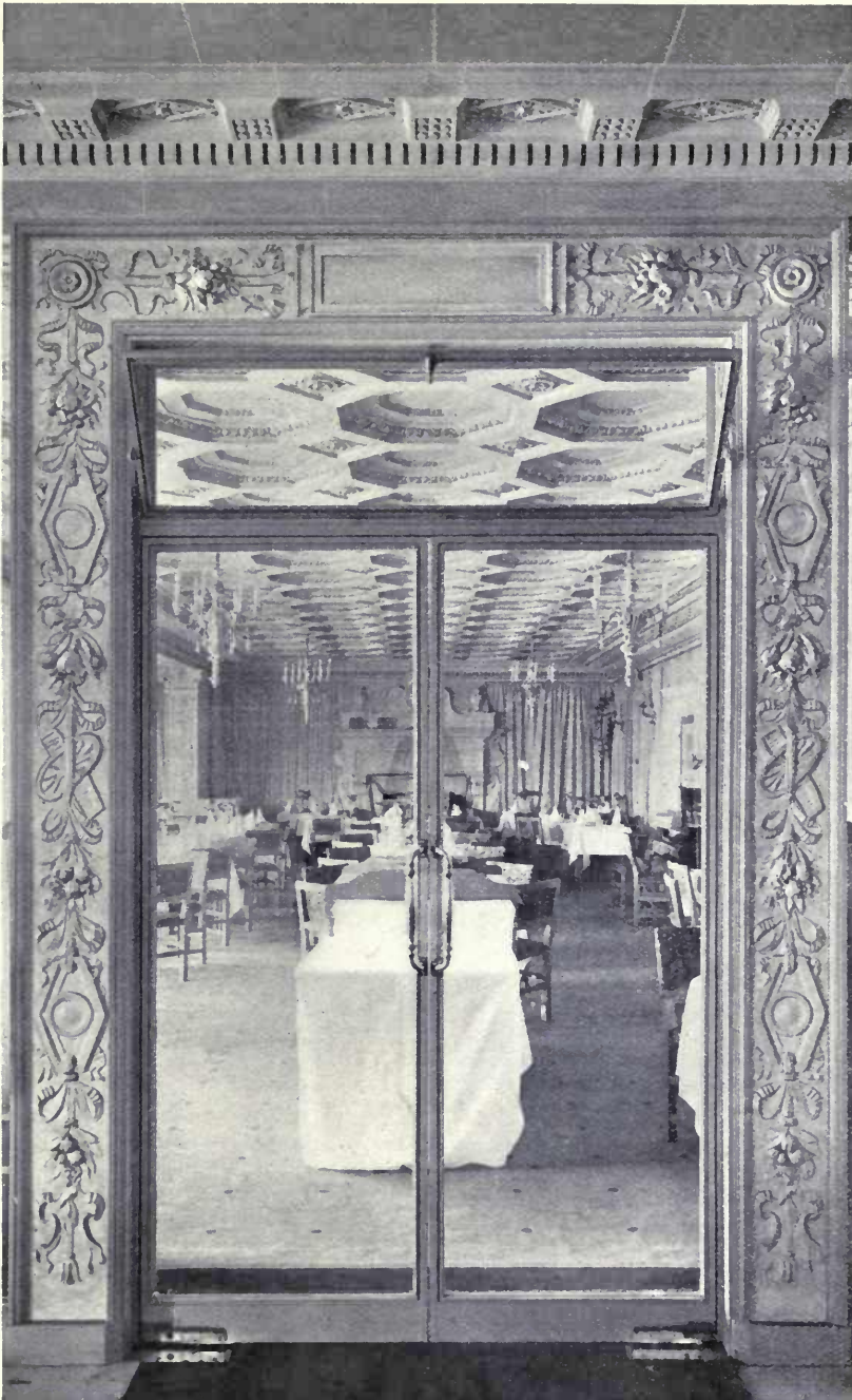
Detail of Italian Restaurant Door from Vestibule.
