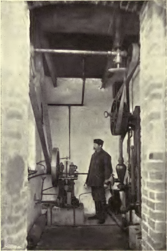
FIG. 219.—ACETYLENE ENGINE WORKING PUMP.
