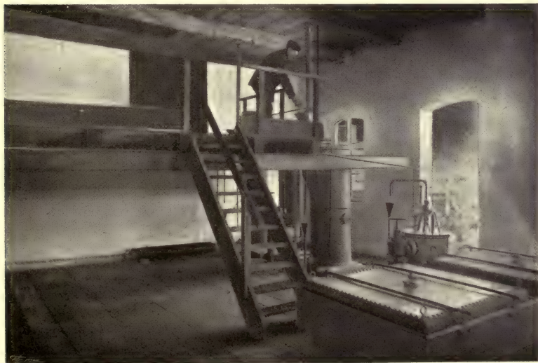
FIG. 135.—INTERIOR OF GENERATOR HOUSE.
