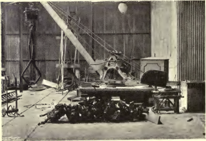
FIG. 68. THE INGOT ROOM AT FOYERS.
