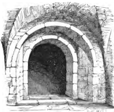
Doorway in Vaults under the Dormitory, Westminster, A.D. 1066.
