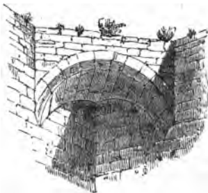
Squinch, Canon's Ashby, Northamptonshire.
