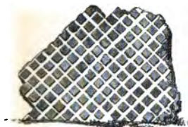
Opus Reticulatum. Net-work. Palace of the Cæsars, A.D. 10.
