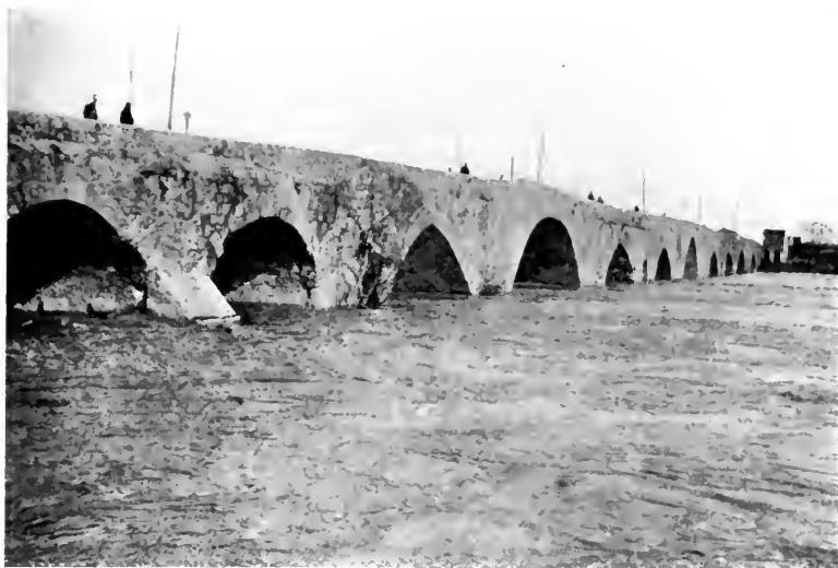
Old Bridge over the Sihon, Adana.
