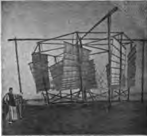
WINDMILLS AT TONG-KU FOR RAISING SALT WATER.
