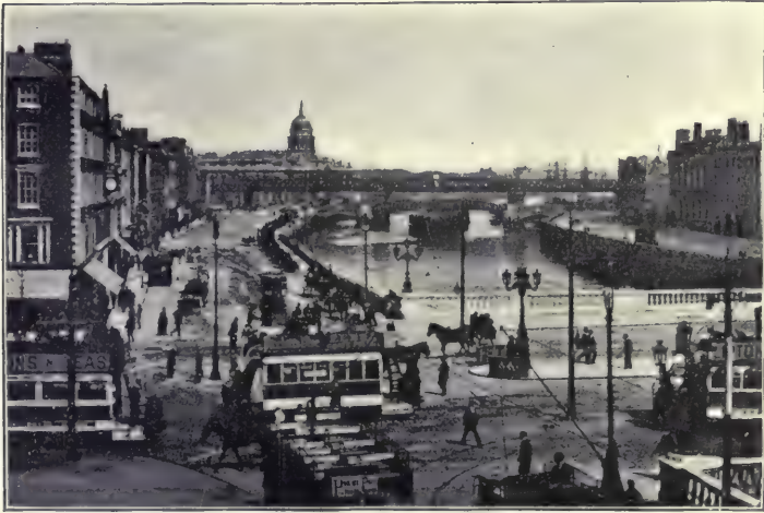
O'Connell Bridge, Dublin.
