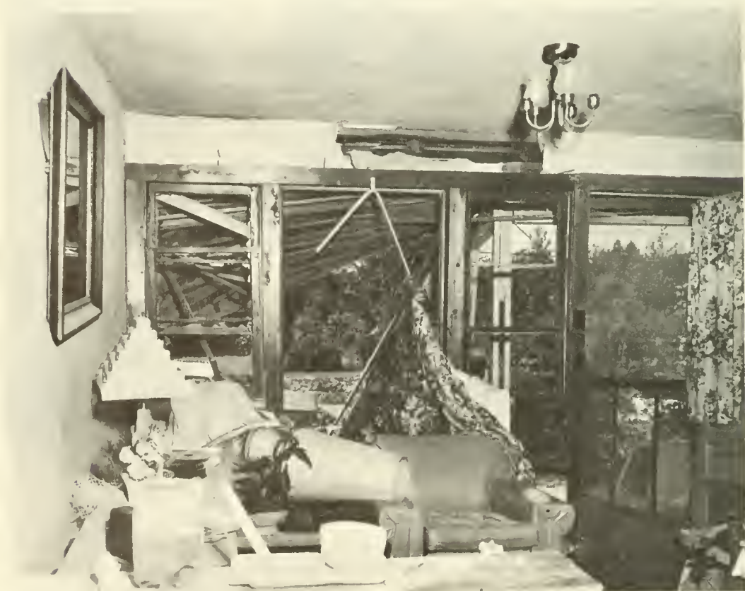
Photographs showing bomb damage to Alyene Quinn residence, McComb, Miss.
