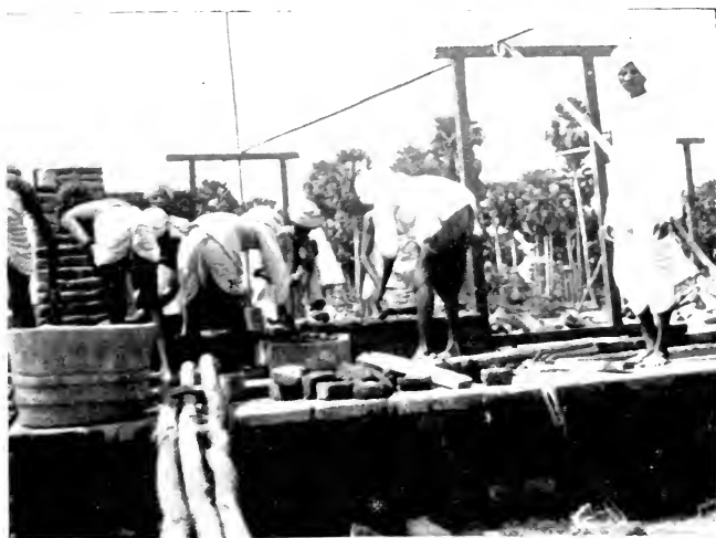
Bricklayers building the new Asylum, Ramachandrapuram.
