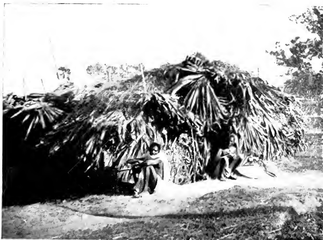
Temporary Huts for lepers. Ramachandrapuram.
