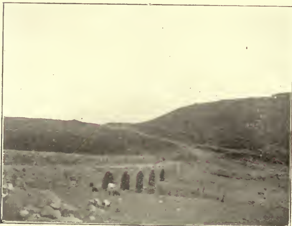
BRIDGE AT DER'AT
