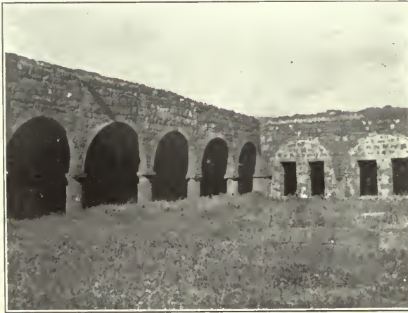
MOSQUE AT EZR'A
