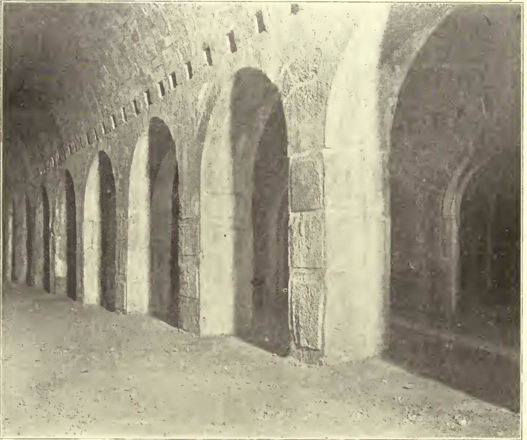
THE UNDERGROUND CONSTRUCTION VULGARLY CALLED SOLOMON'S STABLES
