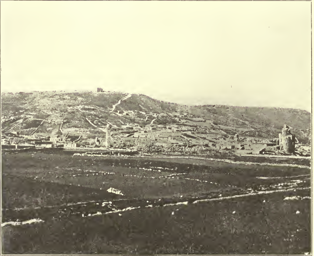
WESTERLY VIEW OF AMMAN
