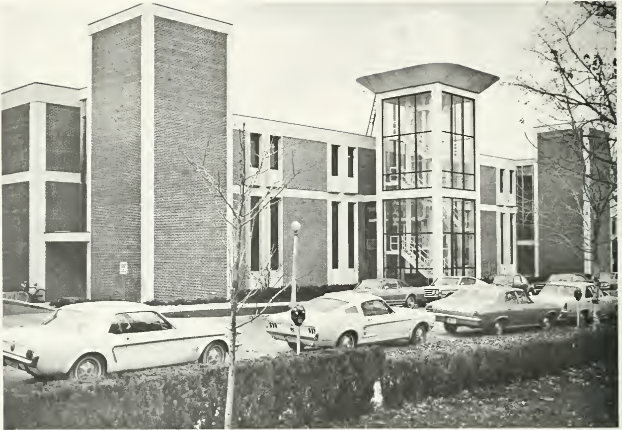
Figure 1. Hydrosystems Laboratory, Home of the Water Resources Center
