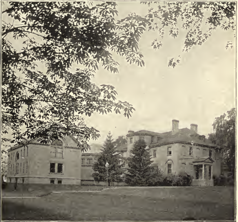
LIBRARY BUILDINGS, NAVAL ACADEMY, ANNAPOLIS
