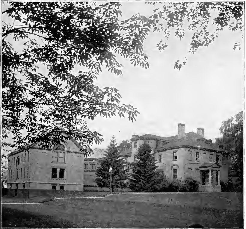
LIBRARY BUILDINGS, NAVAL ACADEMY, ANNAPOLIS
