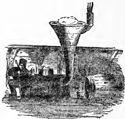
STOVE IN COOK'S GALLEY WITH APPARATUS FOR MELTING SNOW.
