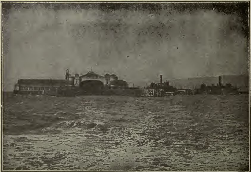
Key route pier—Ferry between Oakland, Berkeley and San Francisco.
